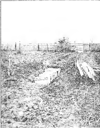
READY FOR THE RAILS
