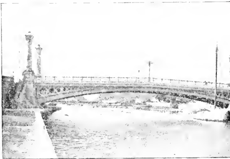
BRIDGE AT MATANZAS.
