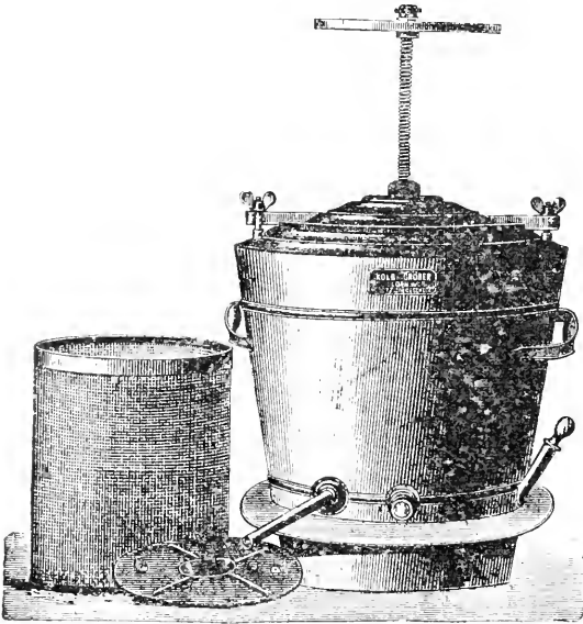
FIG. 14.—KOLB & GROBER STEAM WAX-PRESS.
