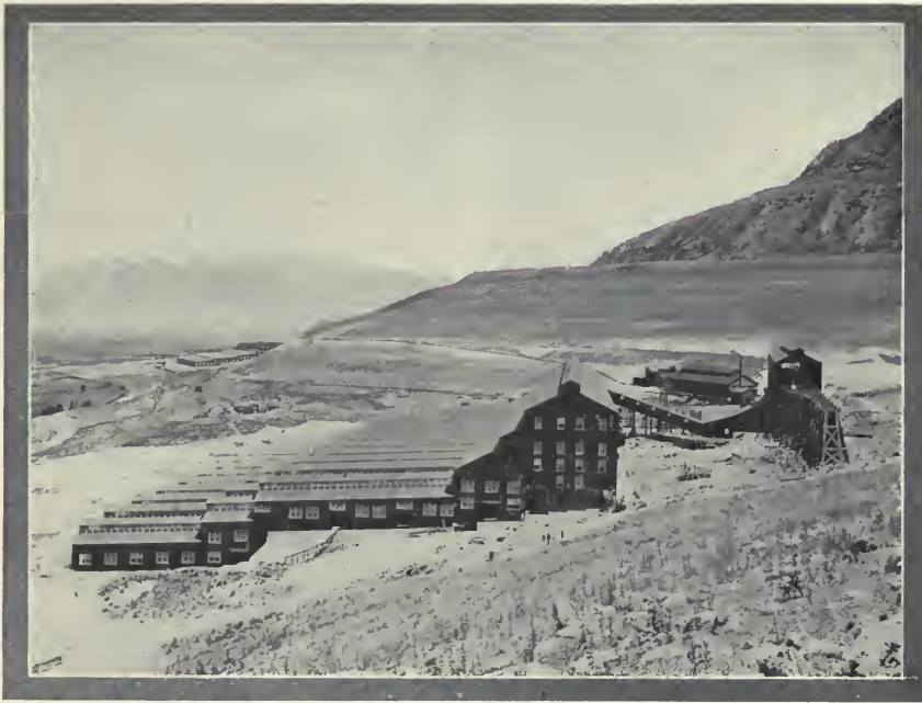
Concentrator Plant, Boston Consolidated Mining Company, Garfield, Utah.
