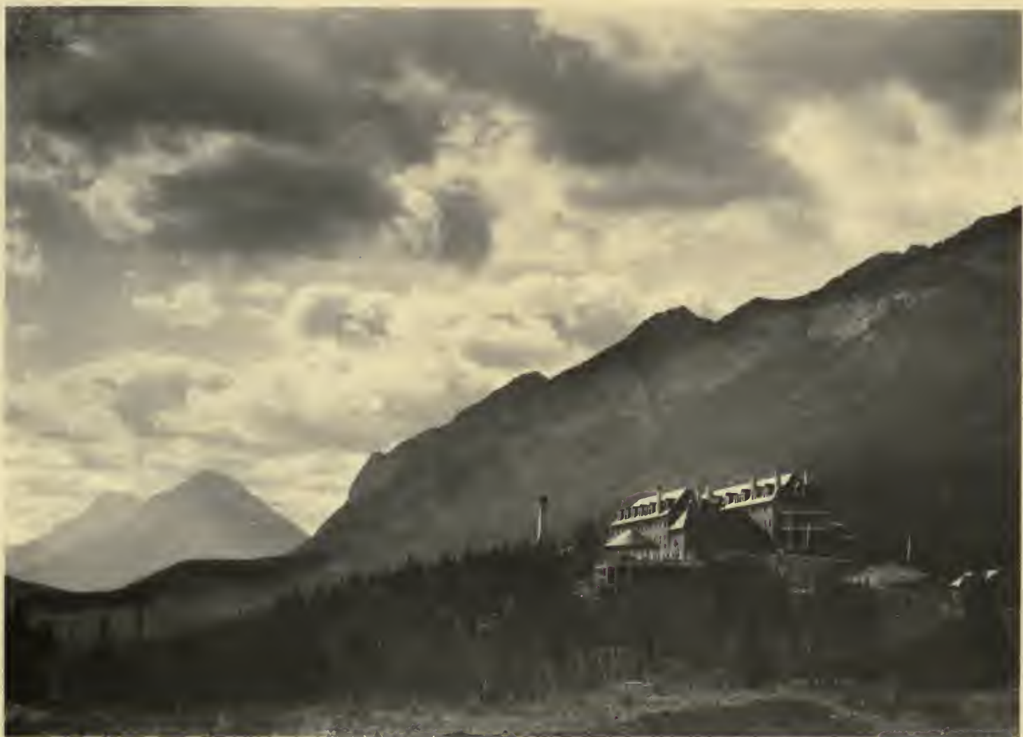
BANFF SPRINGS HOTEL, FROM TUNNEL MOUNTAIN.
