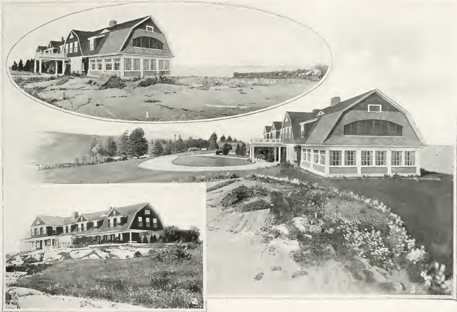
"Weatherend." 1 and 3. The Western Front and Southern End. 2. The Eastern Front and Service End of the House
