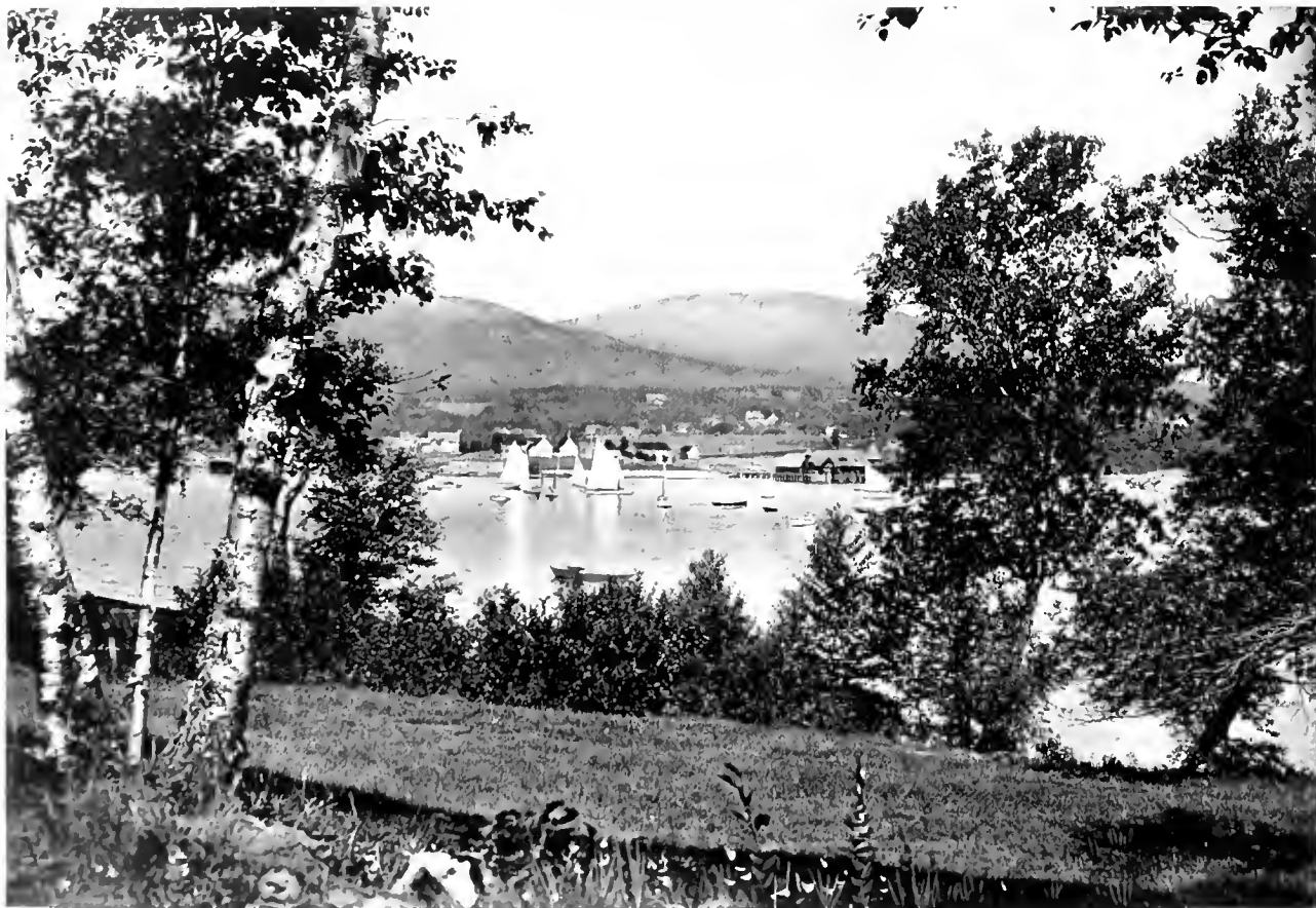
Camden Mountains from Dillingham Point
