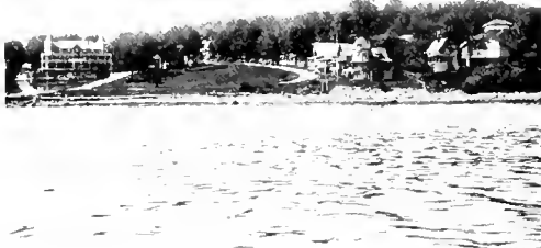
At Northport Northport Inn and Village Green
