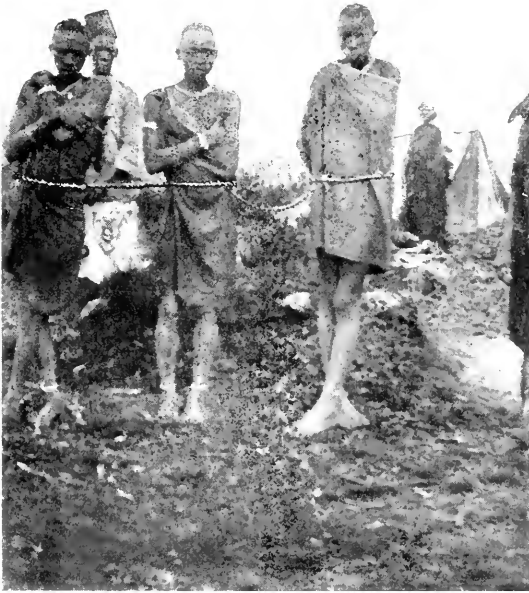
“BARUKU BROUGHT IN THREE PORTERS ROPED TOGETHER”
