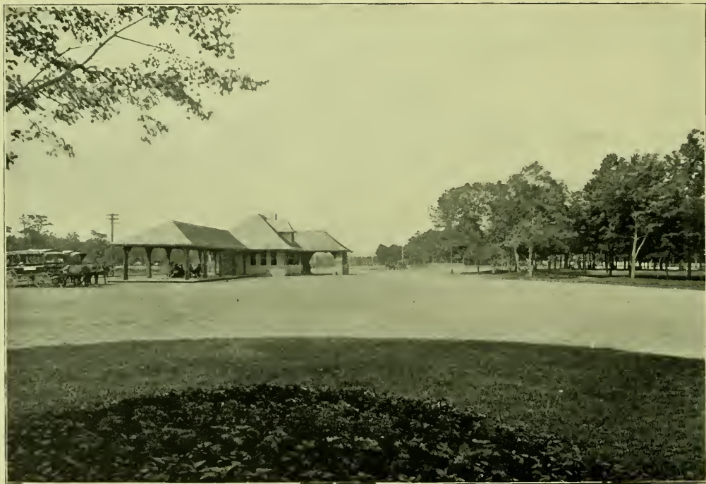
North Asbury Park Station, from the Pennypacker Building.
