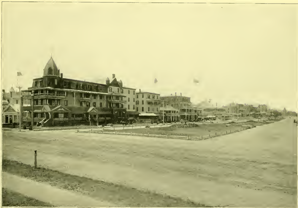
Second Avenue, Looking Southwest from Ocean.
