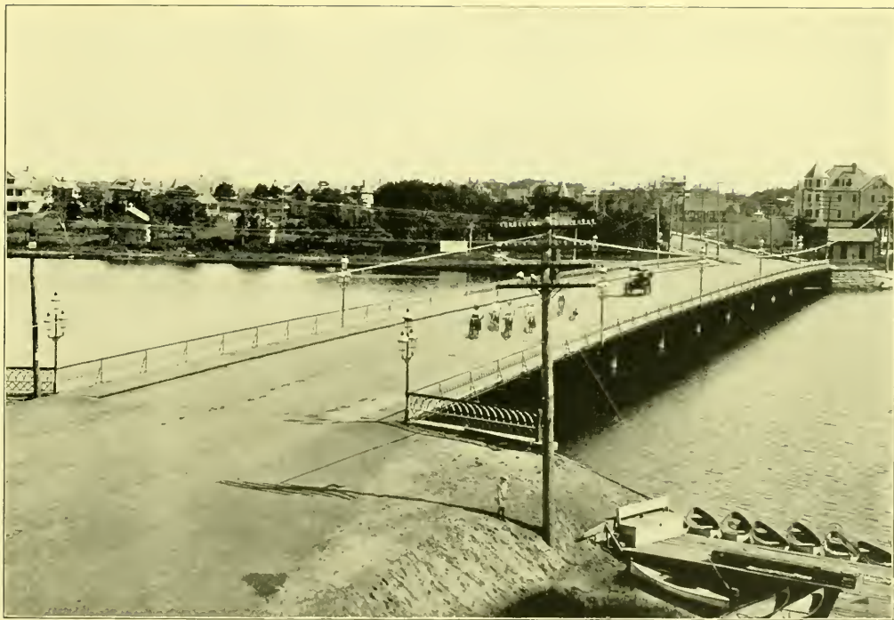
Park Avenue Bridge, Deal Lake, Looking Towards Loch Arbour and Allenhurst.
