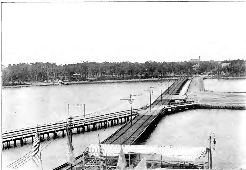
Electric Railroad Bridge across Deal Lake.
