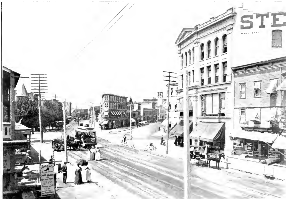
Cookman Avenue, at its Junction with Mattison Avenue and Emory Street.
