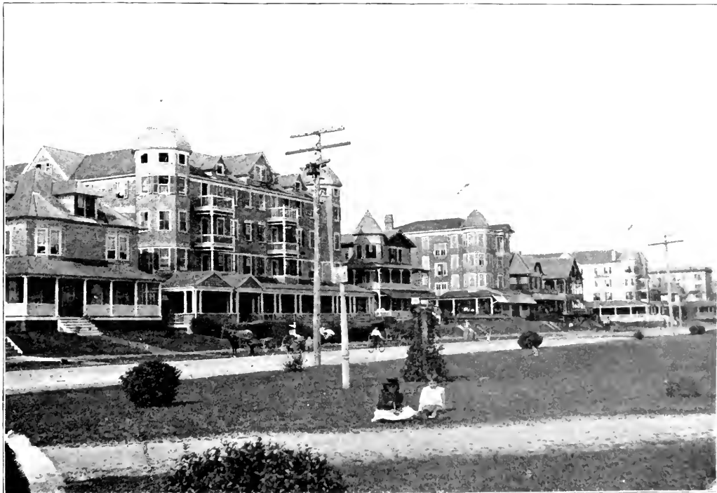
Fifth Avenue. Looking West.
