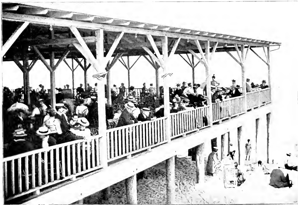
A Corner of the Ross Pavilion.
