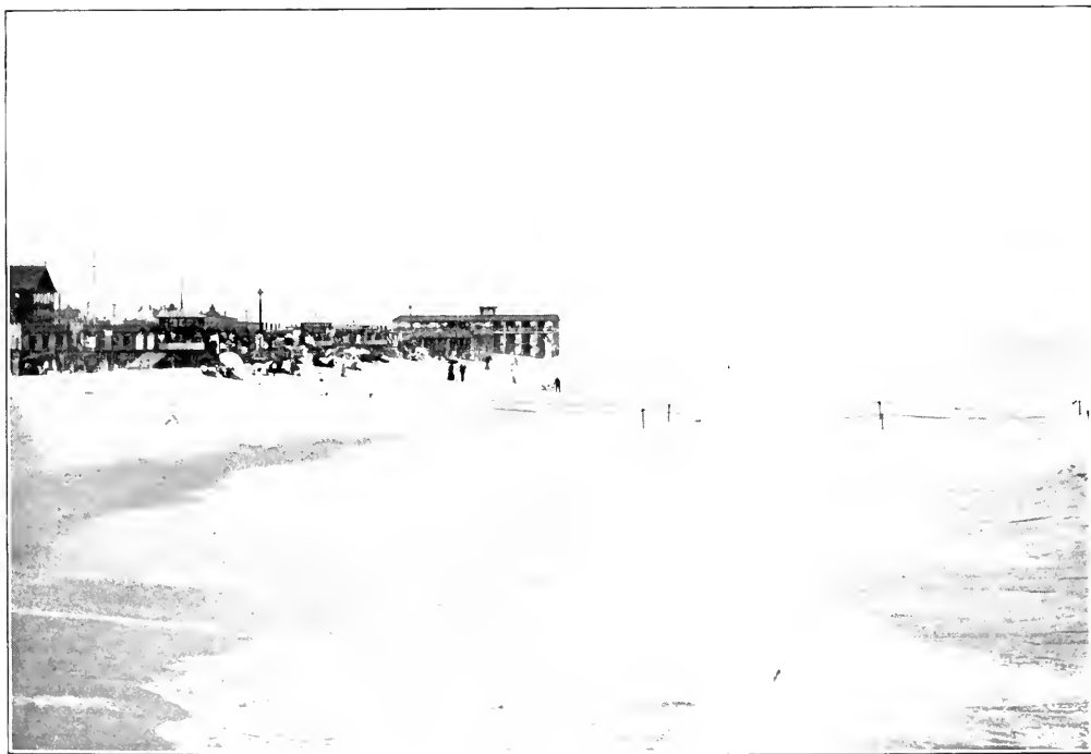
The Beach, Looking North from the Pier.
