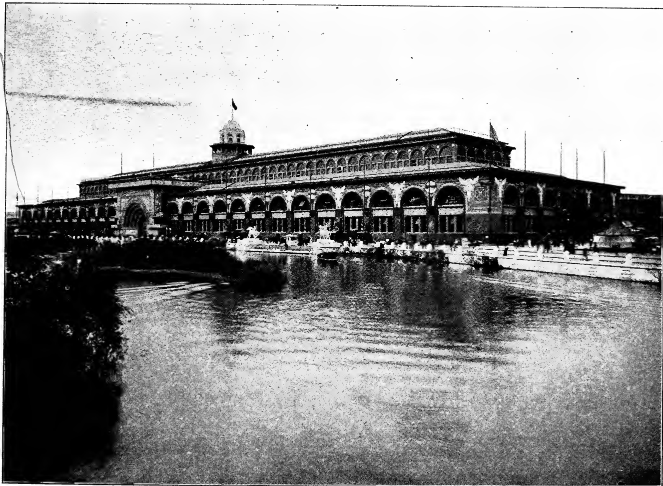
The Transportation Building. —Occupied a ground space of nine acres and the palace itself was 960 x 256 feet; it was decorated in a most sumptuous and novel style and was considered, architecturally, the gem of the Exposition.
