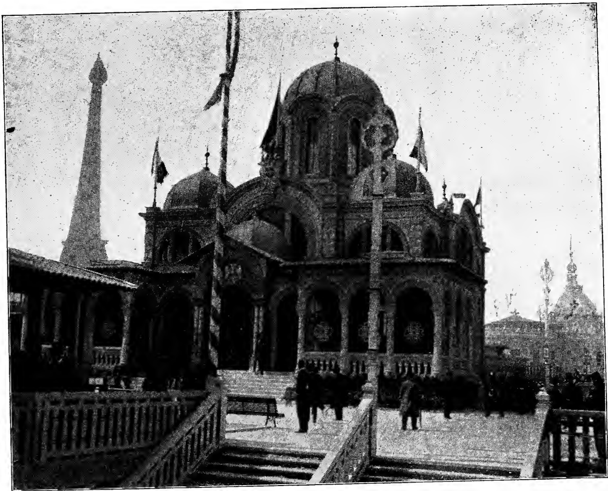
Le Palais Serbe. —At the extreme western end of the Quay of Nations stands the Servian building, a curious mixture of Romanesque and Turkish architecture, very similar to the Greek Building next to it. Serbia is the latest addition to European kingdoms (1882). Area, 19,050 square miles. Population, 2,162,759. King Alexandre Obrenovitch.
