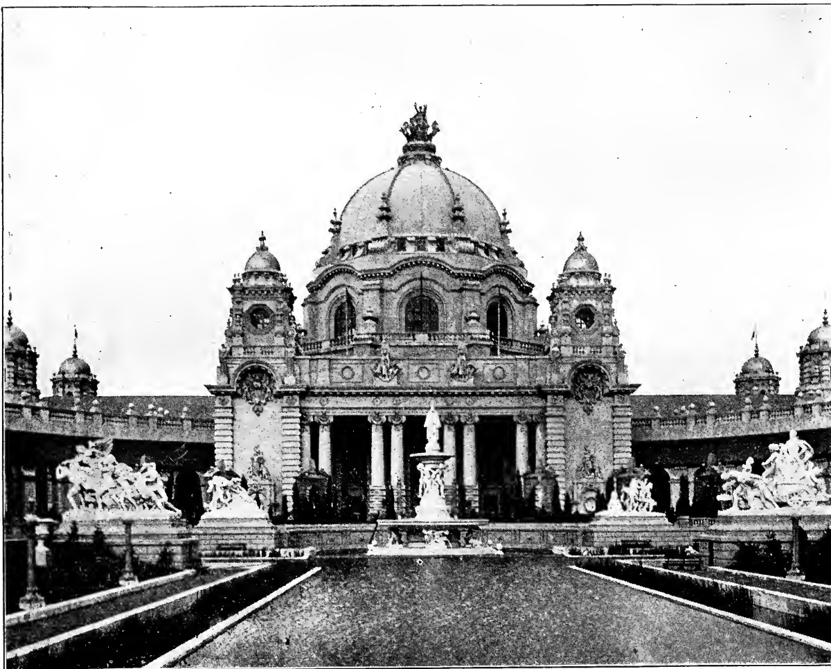
U. S. Government Building. —600 feet long. Congress appropriated $500,000 to be spent upon its group of three buildings and the exhibits therein. It closely resembles the great Cathedral of Mexico City.
