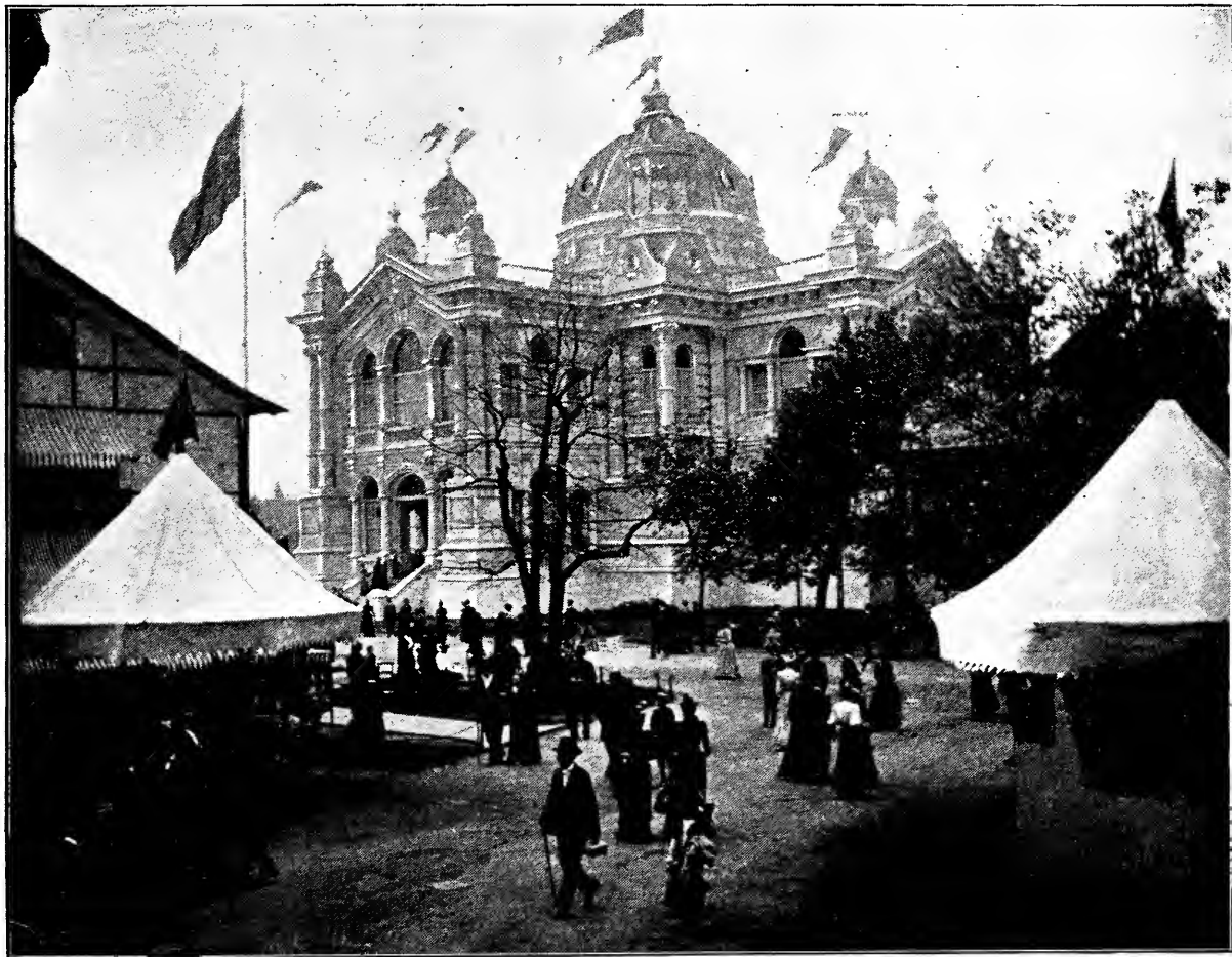
The Brazilian Building. —A very handsome palace, worthy of the largest of the South American republics. The dome was 43 feet high above the rest of the structure.
