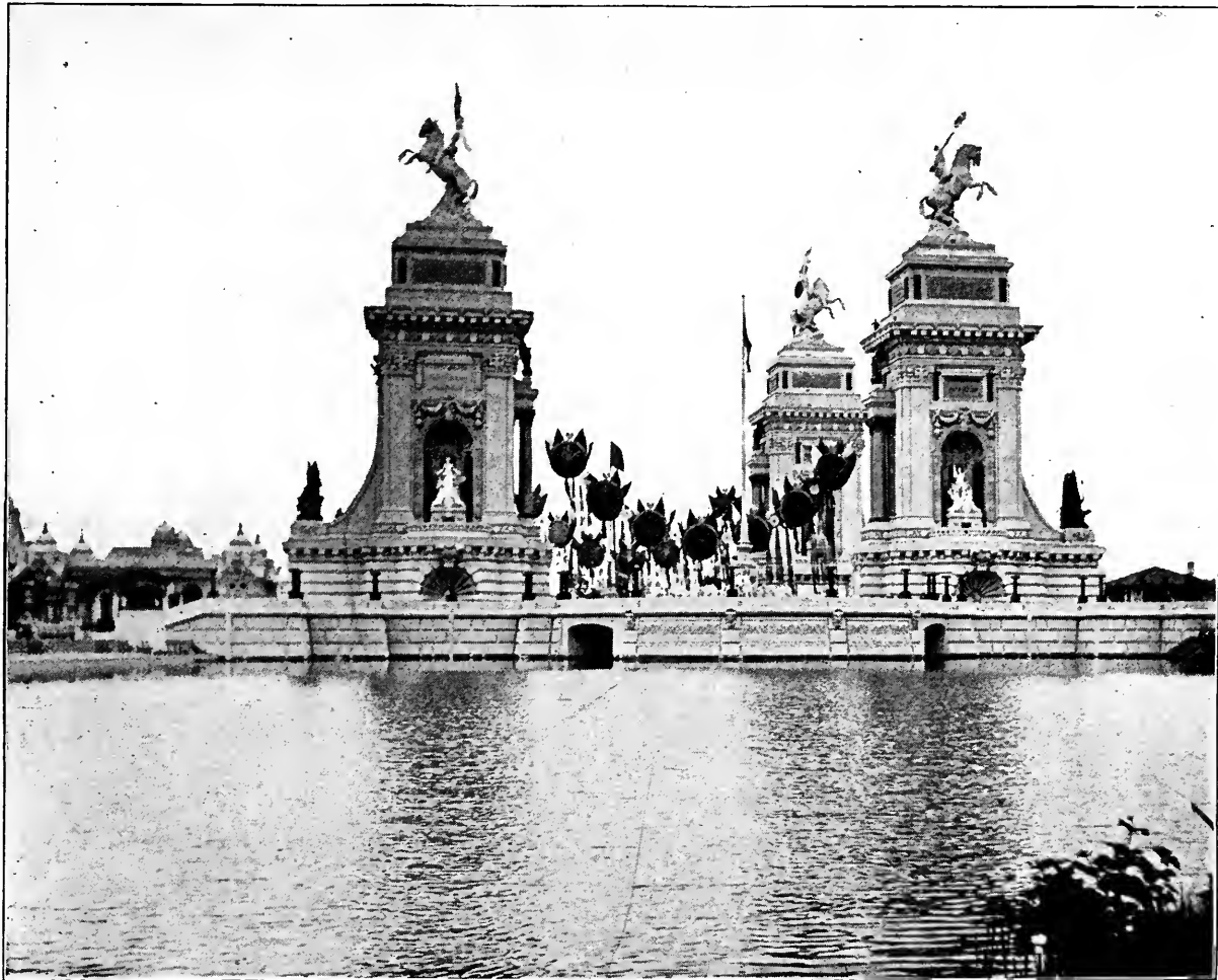
Side View of the Triumphal Causeway. —The horses on the pylons are the largest ever cast. East group is 46 feet high to the top of the standard,
