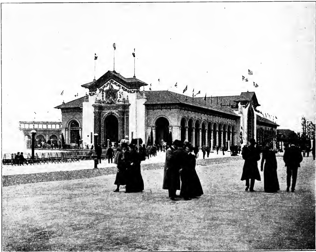
Agricultural Building. —It is 500x150 feet, treated in the style of Spanish Renaissance architecture, and filled with the products of American fields, the suppliers of the world.
