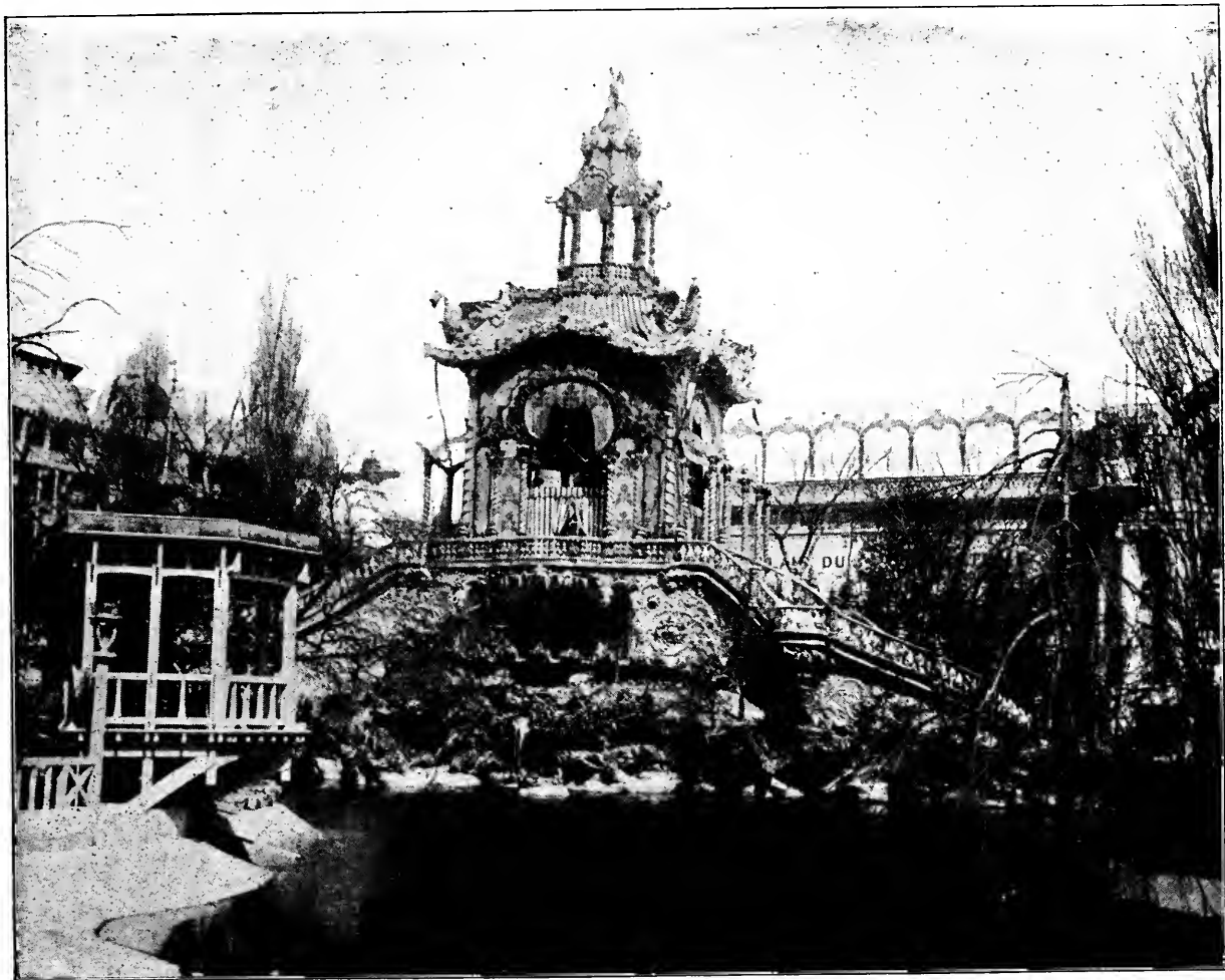
Palais Lumineux. —The LUMINOUS PALACE is made of glass blocks and sheets cemented together; it is 110 feet high and 175 feet in circumference. The stained glass effects by J. A. Ponsin—a famous artist in this specialty, recently deceased—are absolutely unique, electrical light adding to the brilliancy.
