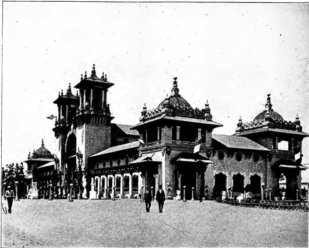
Electricity Building. —This structure is 500 x 150 feet; it is said to contain the largest electrical exhibit ever gathered by this country, which is certainly at the head of the world's progress in that line.
