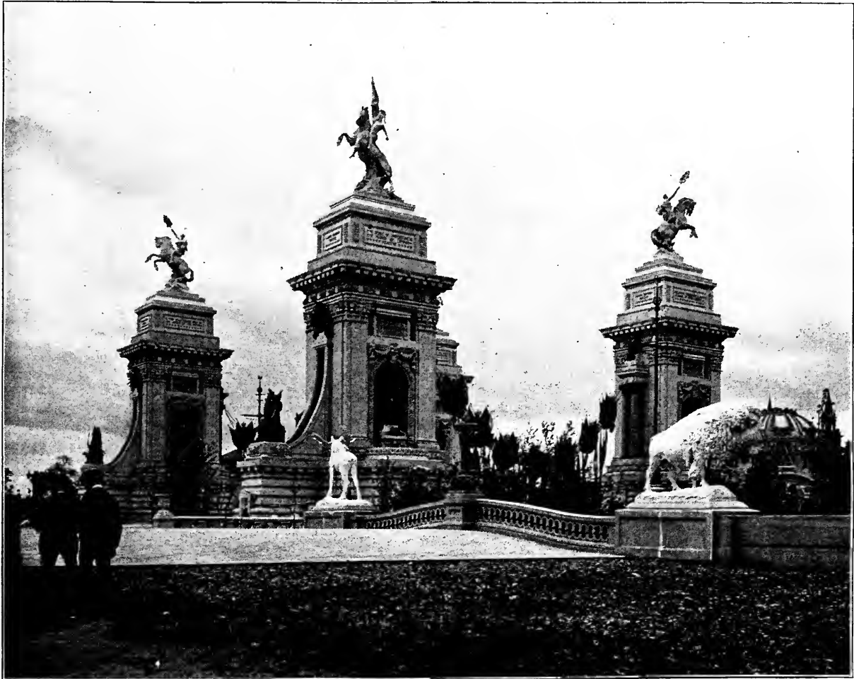
Entering the Triumphal Causeway. —Each of the four Pylons of the Causeway is surmounted by a youth on the back of a horse, 33 feet high, symbolizing liberty's triumph over the trophies of despotism.
