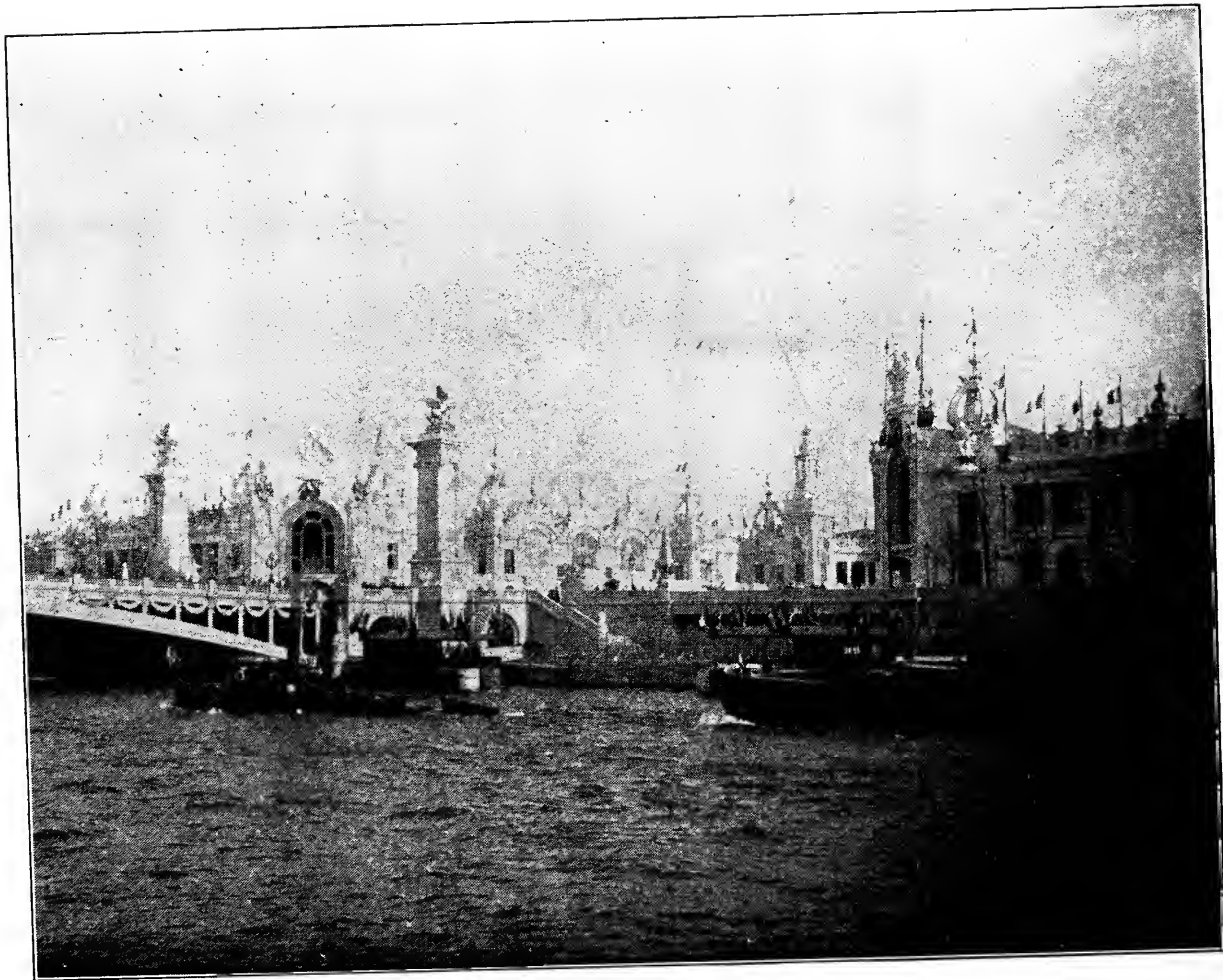
Pont Alexandre III. —The monumental ALEXANDRE III. BRIDGE, just completed, has its southern extremity facing the central avenue of the Esplanade des Invalides, with the PALACES OF VARIED INDUSTRIES. FURNITURE AND DECORATION, on either side, and the Dome of the Invalides at the end.
