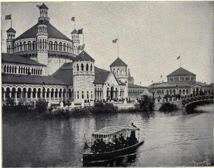
NORTH INLET AND FISHERIES BUILDING.
