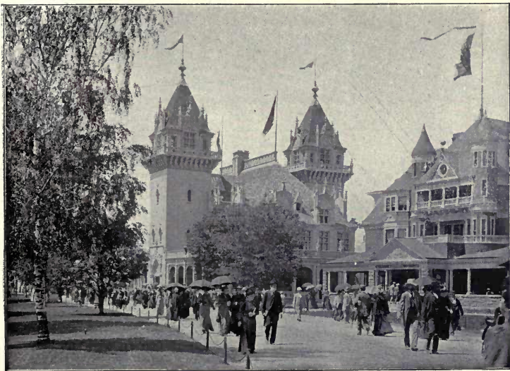
WISCONSIN AND INDIANA STATE BUILDINGS. Wisconsin, 80 by 90 feet, Cost $30,000. Indiana, 100 by 125 feet, Cost $65,000.
