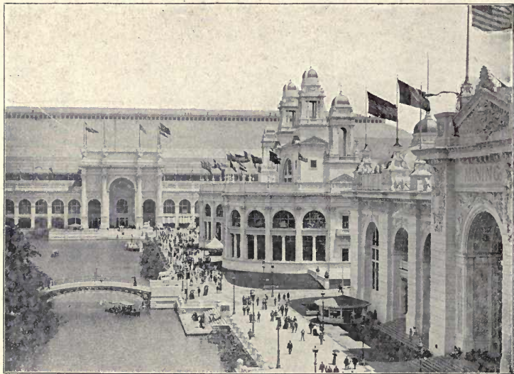
MINING, ELECTRICITY AND WEST ENTRANCE TO MANUFACTURES.
