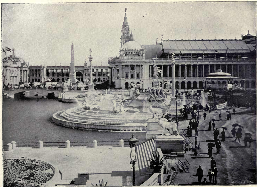
VIEW SOUTH FROM ELECTRICITY BUILDING.
