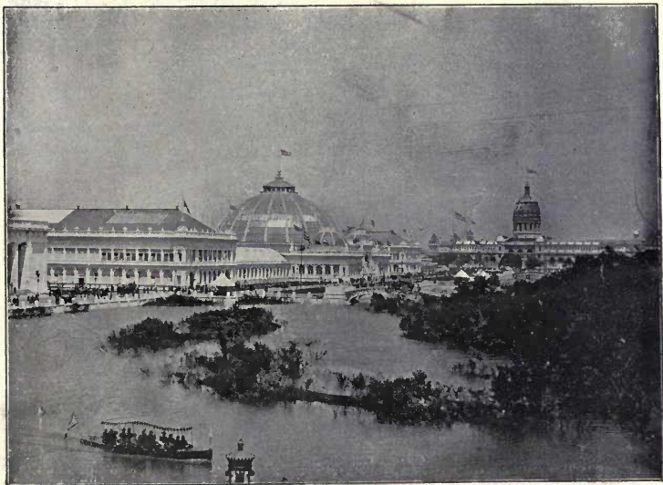
VIEW FROM NORTH END OF ELECTRICITY BUILDING.
