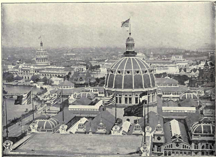
NORTH FROM ROOF OF MANUFACTURES BUILDING.
