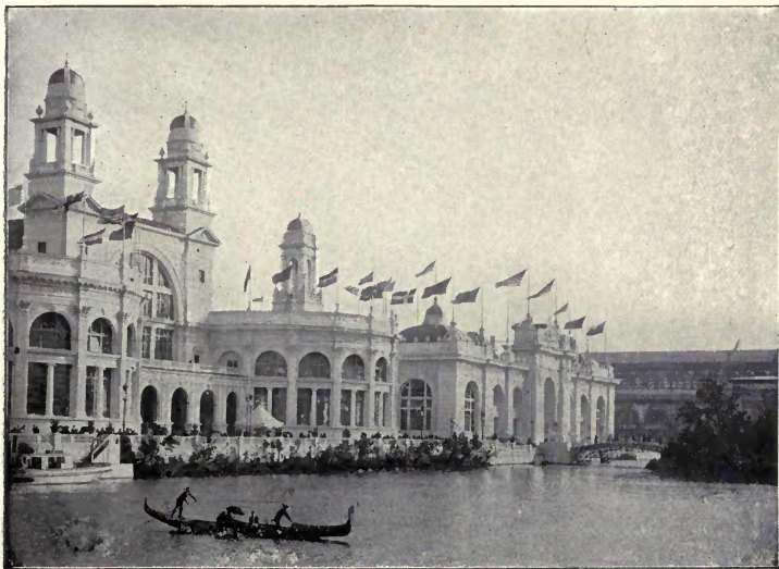
NORTH END OF ELECTRICITY AND MINES AND MINING BUILDINGS.
