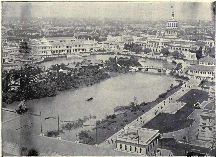
NORTHWEST FROM ROOF OF MANUFACTURES BUILDING.
