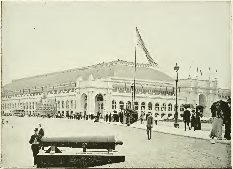
MANUFACTURES BUILDING FROM LAKE SHORE.
