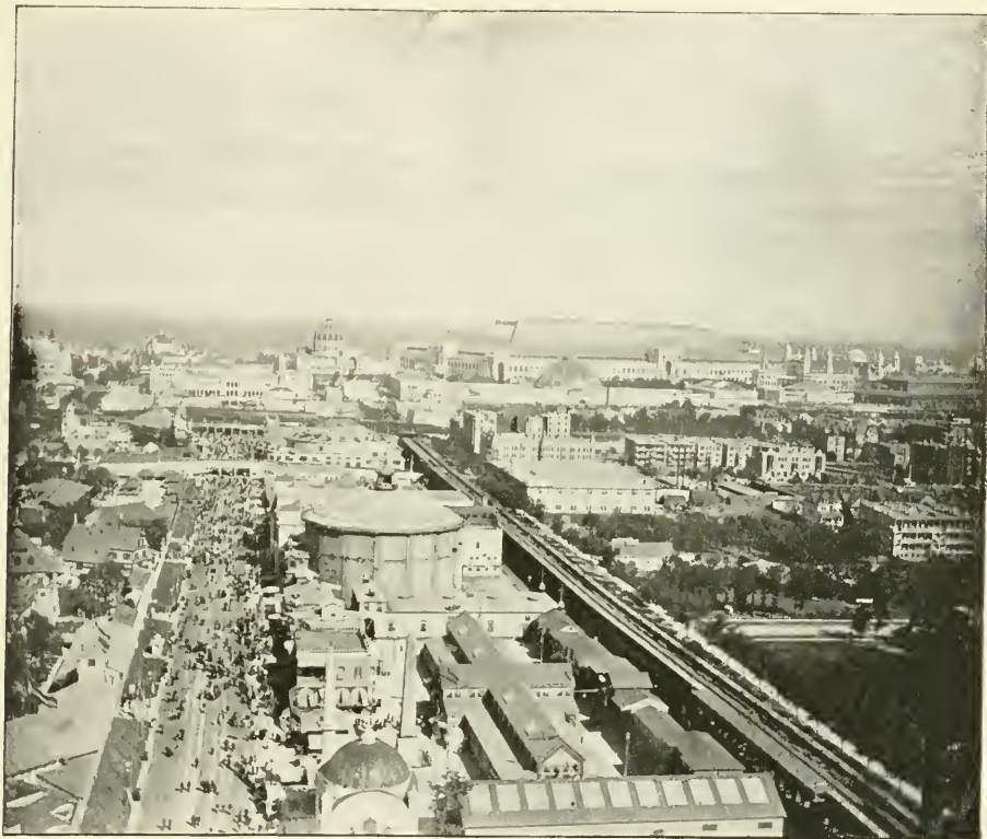
LOOKING SOUTHEAST FROM FERRIS WHEEL.
