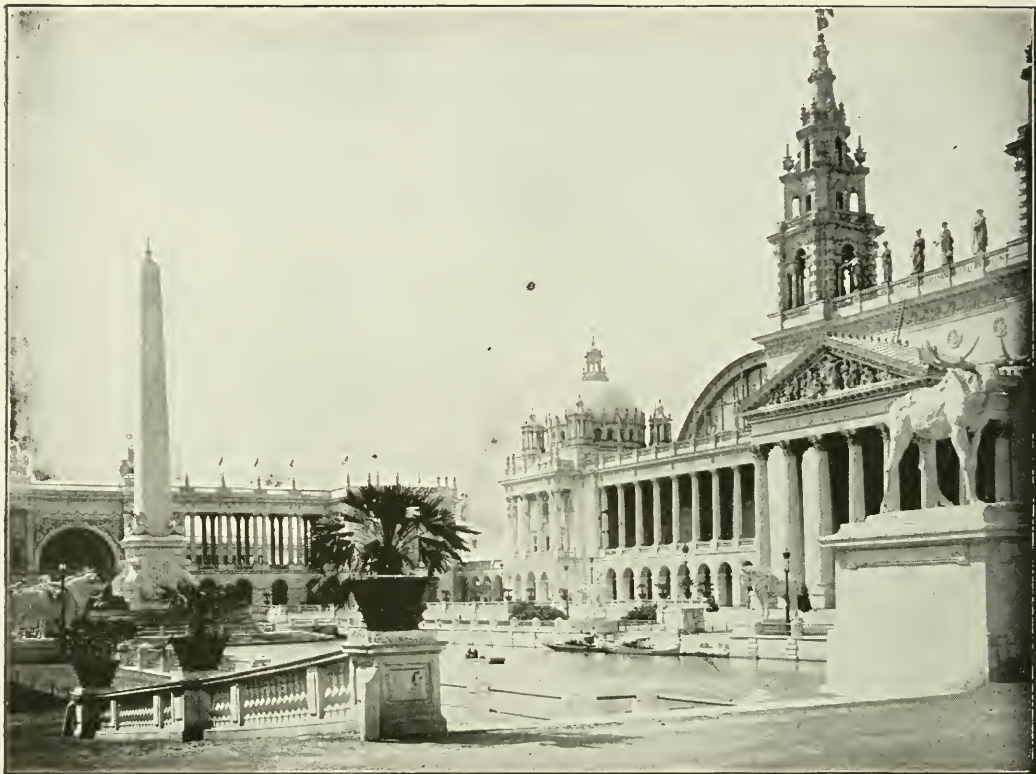
EAST END OF MACHINERY HALL AND COLONNADE.
