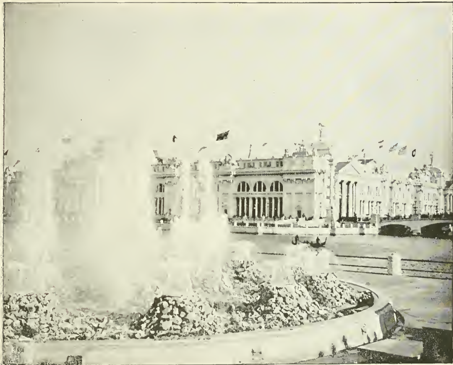
DETAIL OF ELECTRIC FOUNTAIN.
