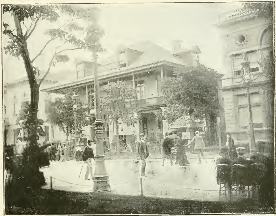
LOUISIANA STATE BUILDING.
