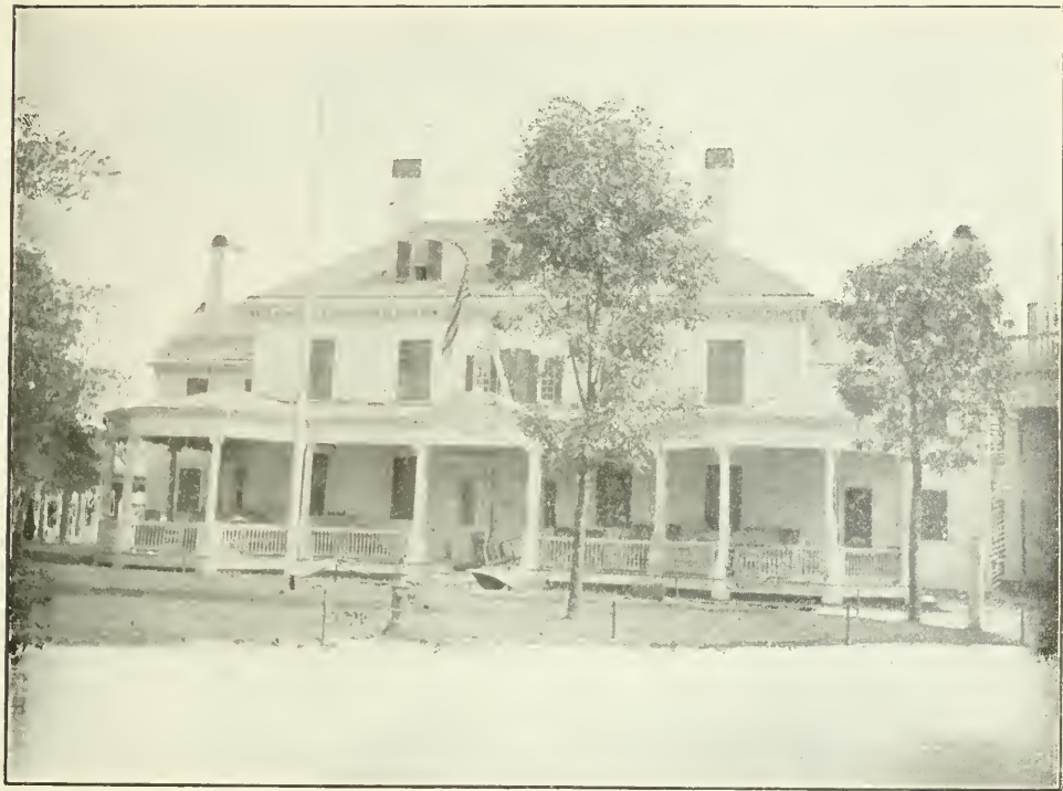
NEW JERSEY STATE BUILDING.
