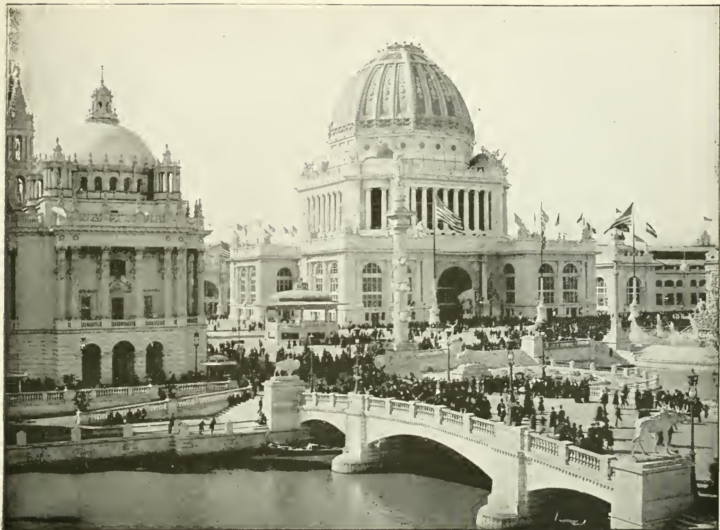
ADMINISTRATION BUILDING FROM AGRICULTURE.
