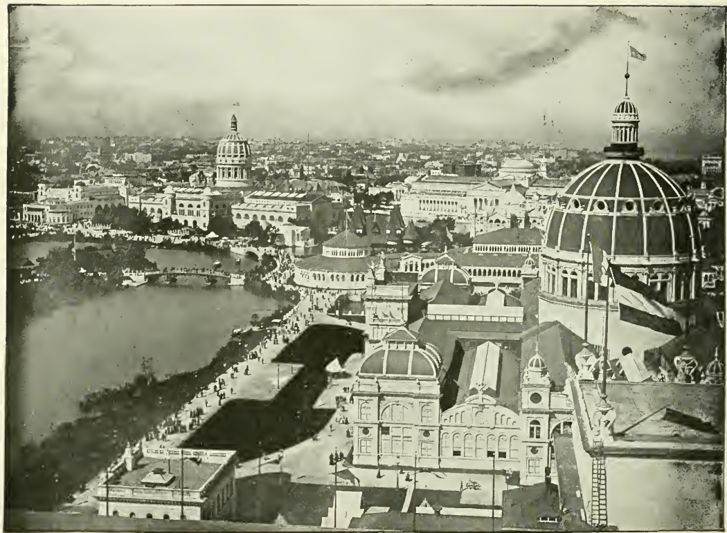
NORTHWEST FROM ROOF OF MANUFACTURES BUILDING.
