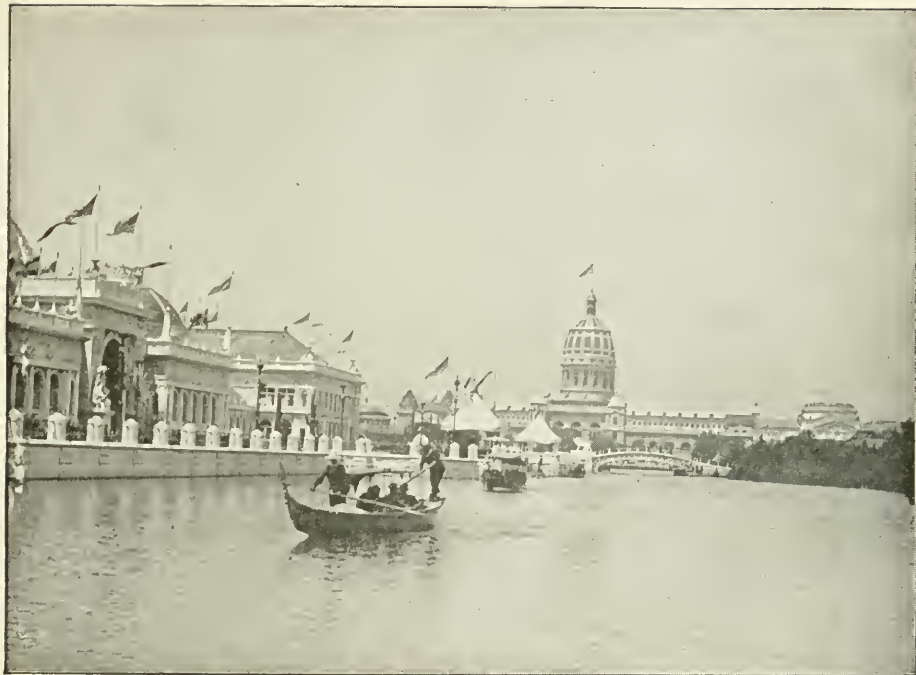
NORTH FROM BRIDGE SOUTH OF HORTICULTURAL BUILDING.
