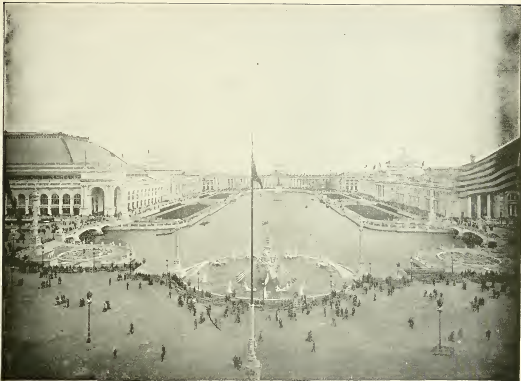
VIEW EAST FROM GALLERY OF ADMINISTRATION BUILDING.
