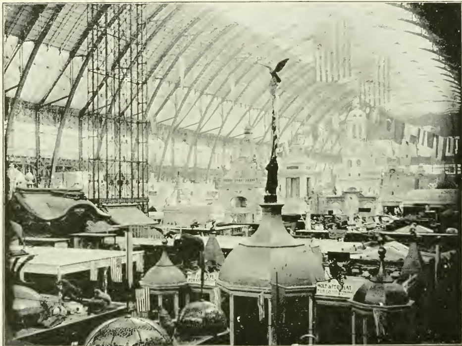
INTERIOR VIEW OF MANUFACTURES BUILDING.
