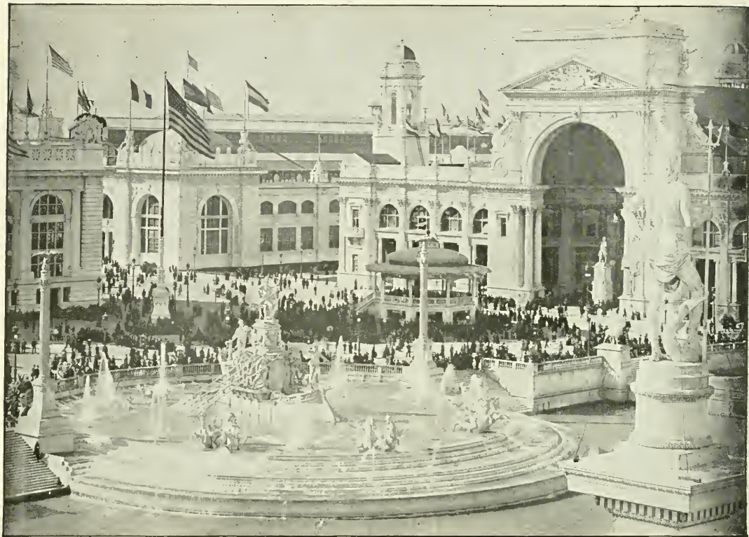
VIEW NORTHWEST FROM AGRICULTURAL BUILDING.
