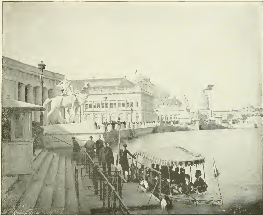
VIEW NORTH FROM LANDING AT TRANSPORTATION BUILDING.
