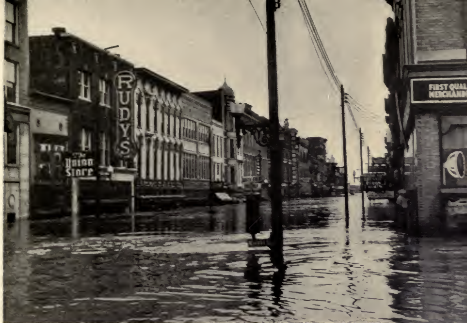
WATER DAMAGE: WHEN THE FLOODS CAME TO PADUCAH
