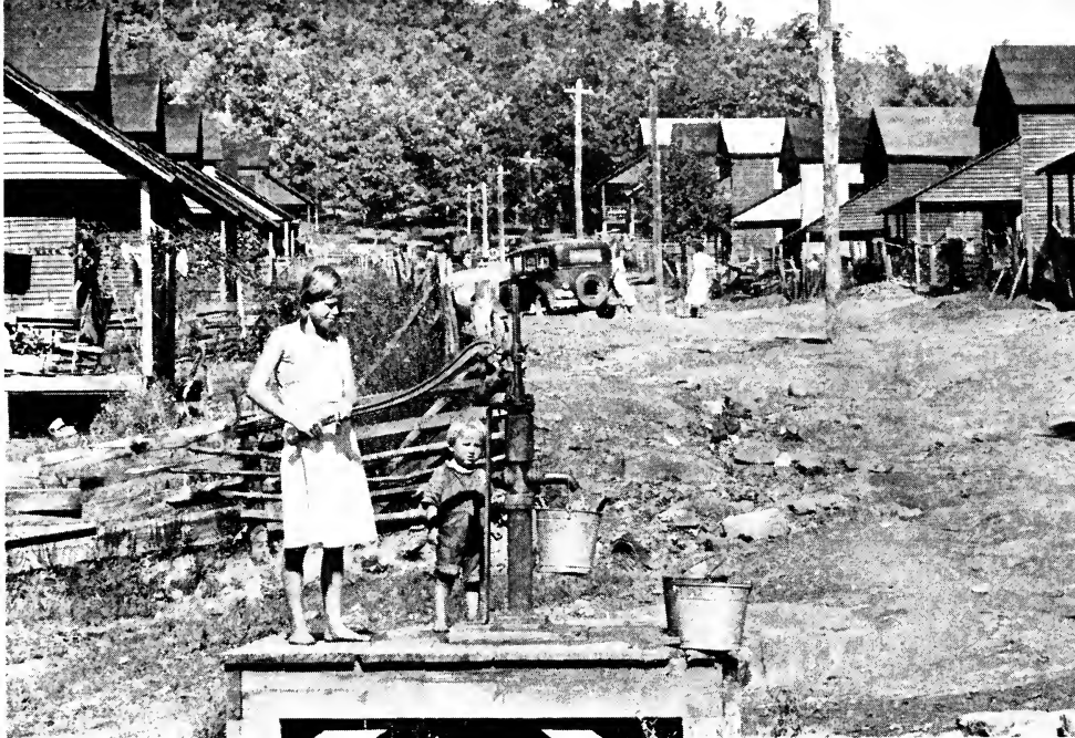
THIS TOWN'S OUT-OF-WORK MINERS HELPED BUILD DAMS
