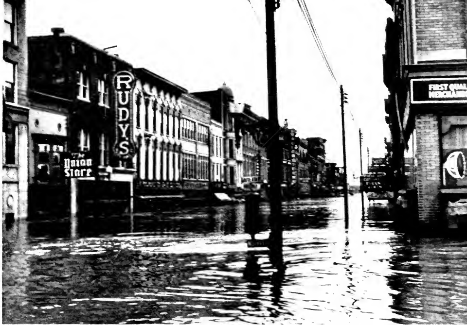
WATER DAMAGE: WHEN THE FLOODS CAME TO RADUCA—
