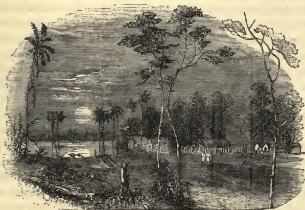
AT THE DIGGINGS.
