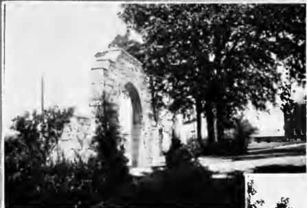
ONE OF THE ARCH ENTRANCES
