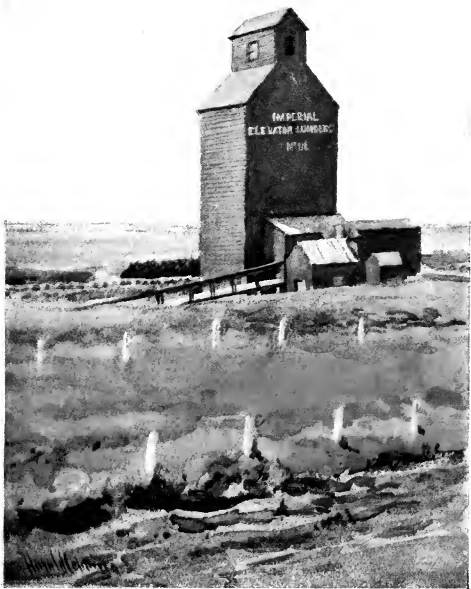
“NOTHING THEN REMAINS BUT FOR HIM TO DRIVE HIS WAGON-LOADS OF WHEAT TO THE NEAREST ELEVATOR” (PAGE 43). THESE USEFUL, IF UNPICTURESQUE, STRUCTURES ARE CONSPICUOUS LAND-MARKS IN ALL SETTLED DISTRICTS OF THE PRAIRIE PROVINCES.
