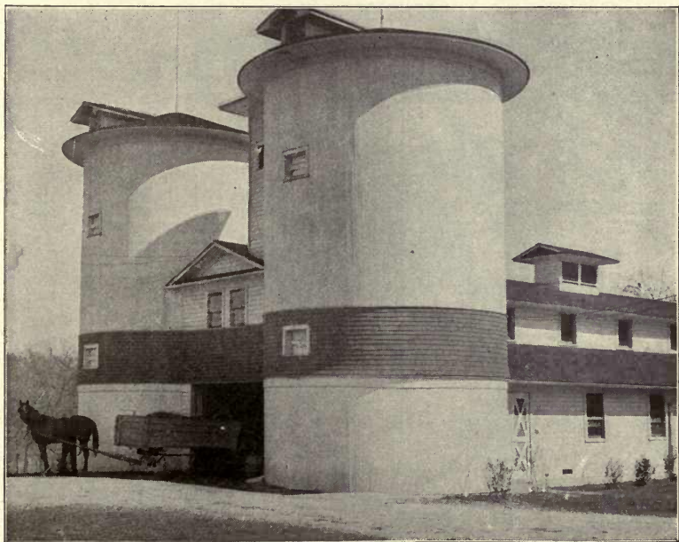
Two wood silos, one lined with vitrified brick and the other with lath and plaster
