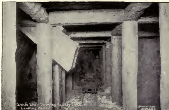
Square-Sets, Gold Coin Mine, Cripple Creek, Colorado.
