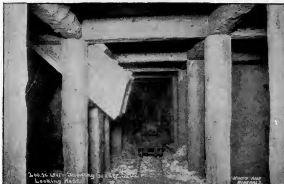
Square-Sets, Gold Coin Mine, Cripple Creek, Colorado.
