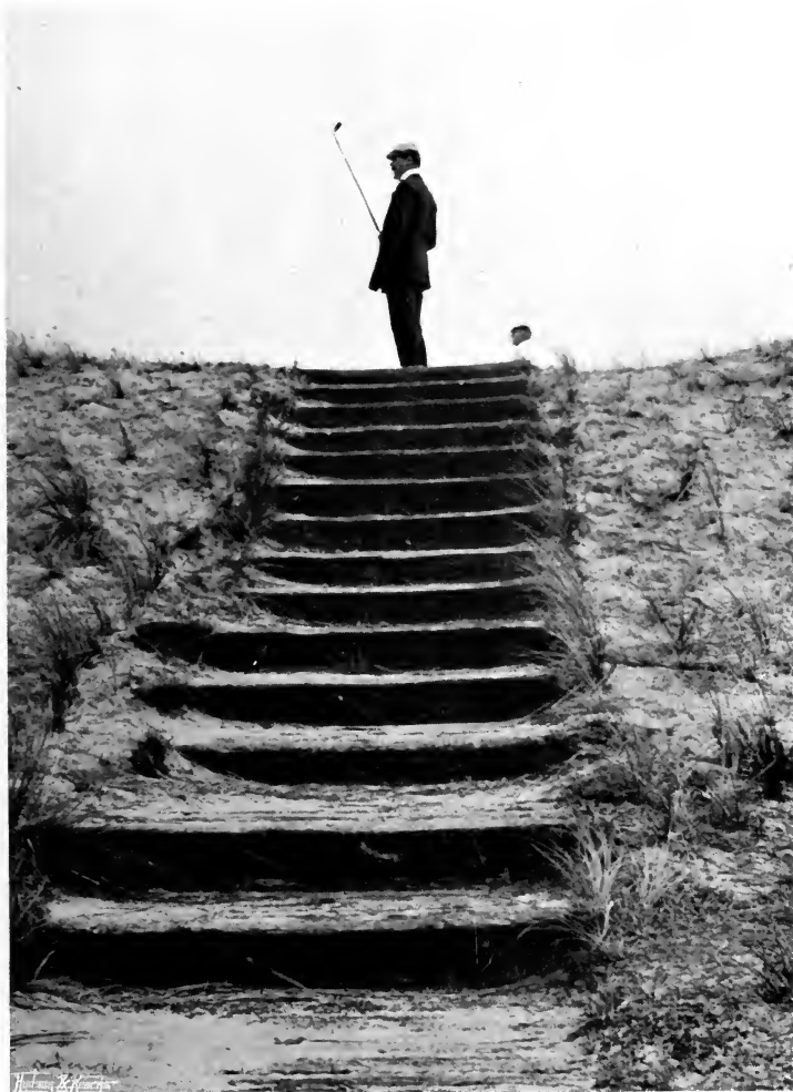
STEPS IN BUNKER (TO SAVE SAND BLOWING).
