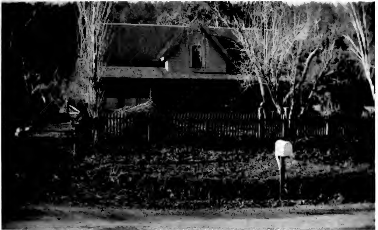
This view of the house, taken before 1937, shows that the eaves decoration has been altered and the south side of the porch has been enclosed. The picket fence would soon be removed. Courtesy of Henrietta Greer.
