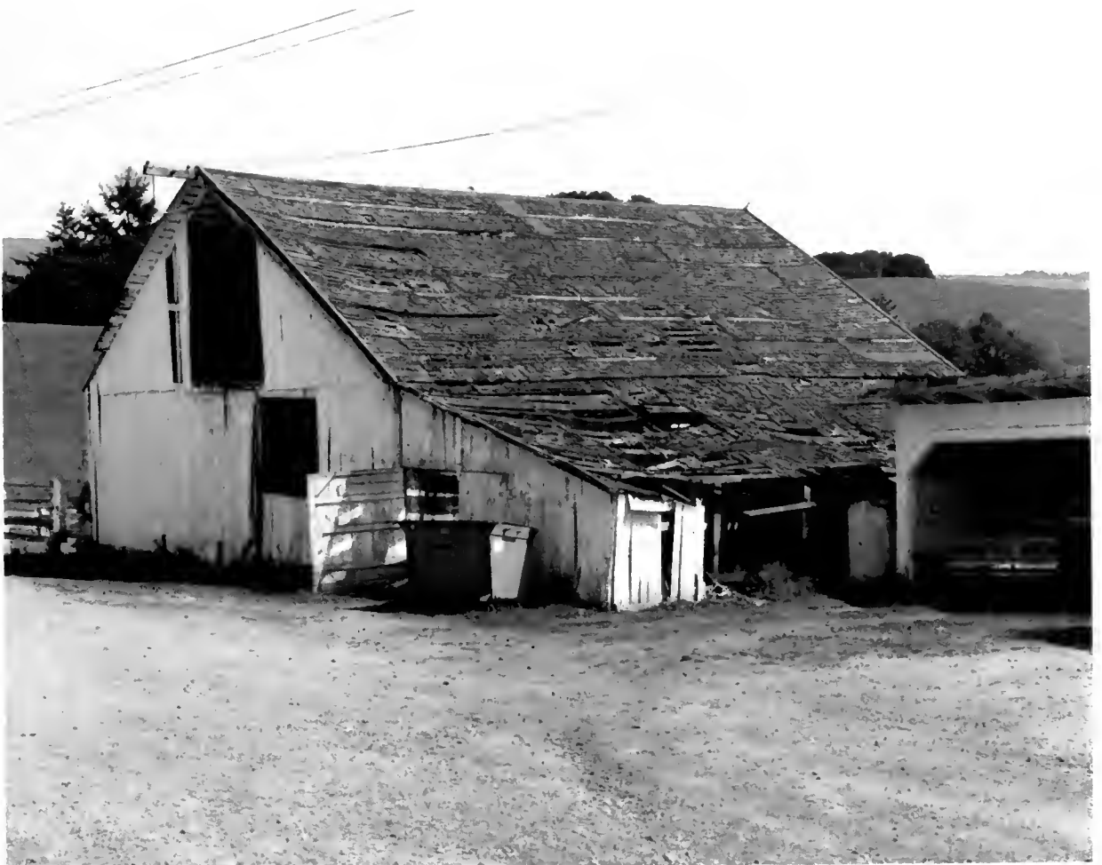
The Truttman Ranch horse barn as it appeared in 1990; the carriage shed is at the right. These and many of the surrounding structures were torn down in 1994. NPS photograph by Dewey Livingston.
