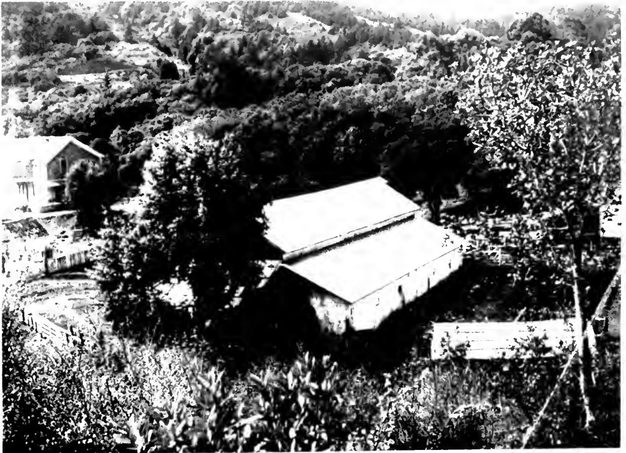
The McCurdy Ranch, looking west/northwest, around 1915. Note the house at far left. Courtesy of the DeFraga family.
