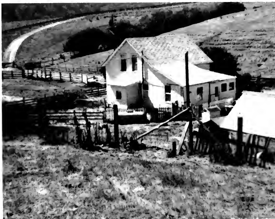
View of the Bordessa Ranch house before it was remodeled. Courtesy of Virginia (Bordessa) McFadden.
