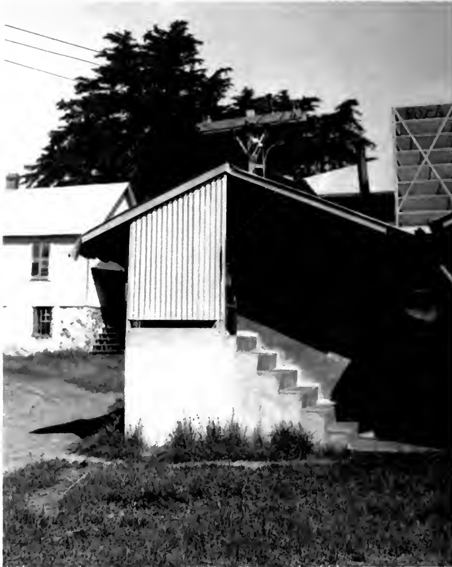
The milk room of the Grade A dairy barn at Wilkins Ranch as it appeared in 1943. The stairs led to the hopper where the fresh milk was poured for cooling before shipment; the cooling tower is visible in the right rear. Courtesy of Roy Farrington Jones.
