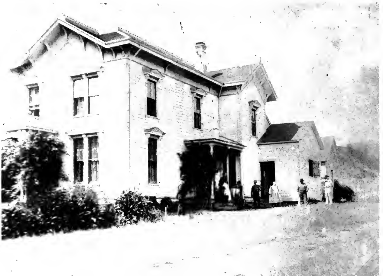
The Randall house, circa 1890-1900. Note that the chimney has been removed and fish scale shingles have covered the south wall. Bancroft Library.
