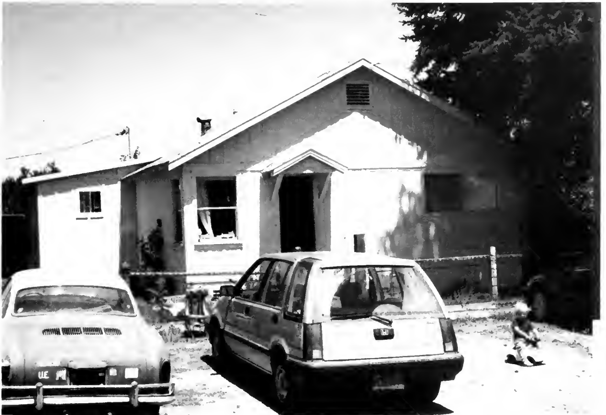
The small 1944 house as it appeared in 1990. The house was later burned for fire training. Photo by Dewey Livingston.
