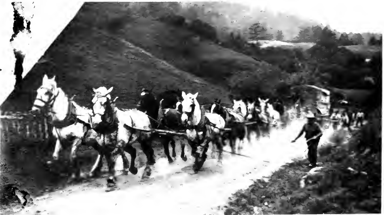
A load of equipment for the Marconi Wireless station at Bolinas is hauled from the train depot at Point Reyes Station up Muscio Hill in 1914. Courtesy of Helen Harris.
