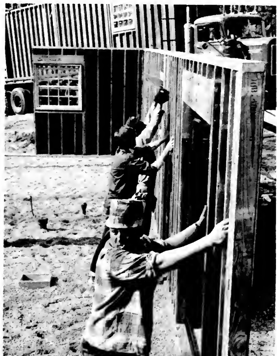
Pre-fab house being erected in Maryland.
