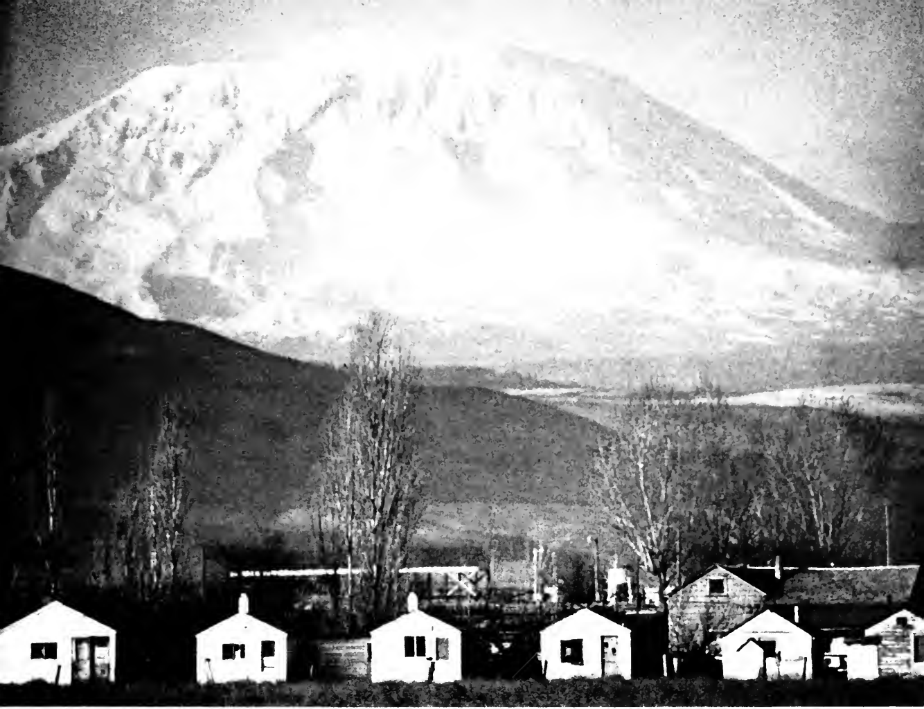
Farm labor housing near Granger, Wash.
