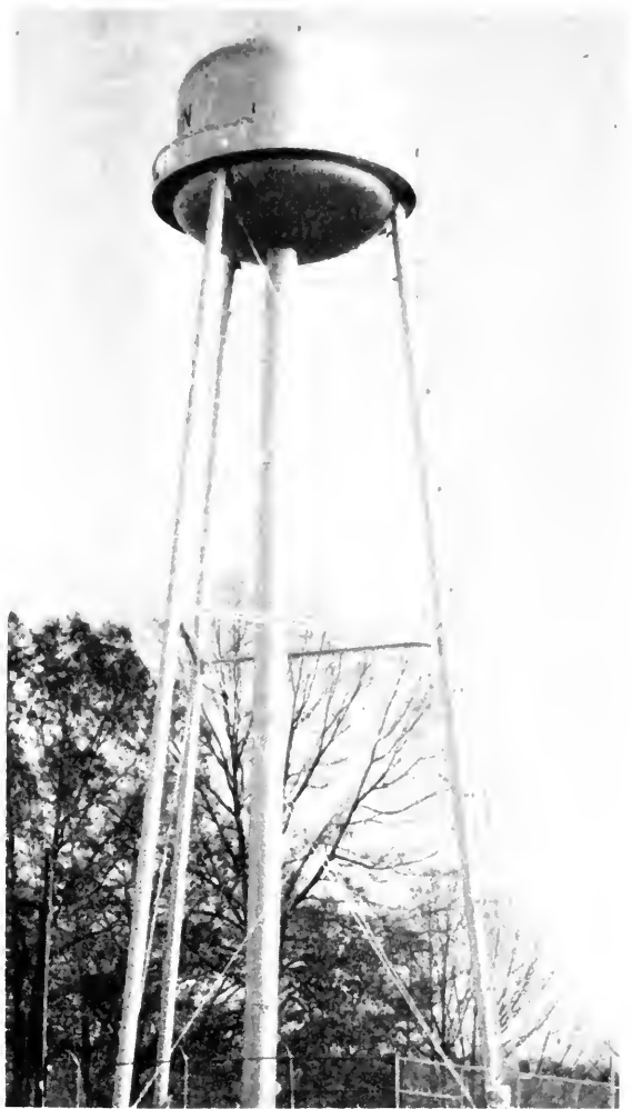
Water tower in Warren County, Tenn.
