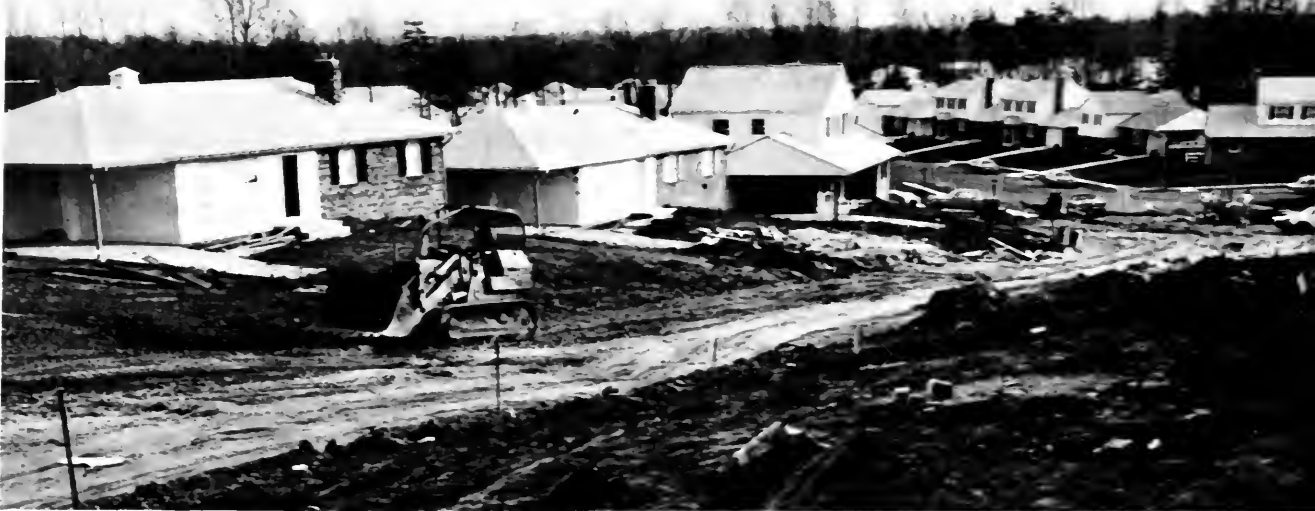
Construction of new homes near Largo, Md., a suburb of Washington.
