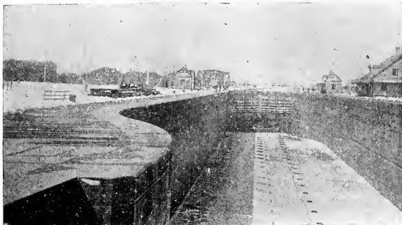
INTERIOR OF THE PRESENT LOCKS, PUMPED DRY FOR REPAIRS.
