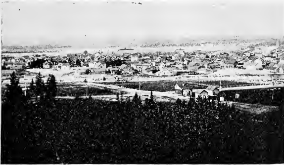
THE SOO AS SEEN FROM CHANDLER'S HILL.
