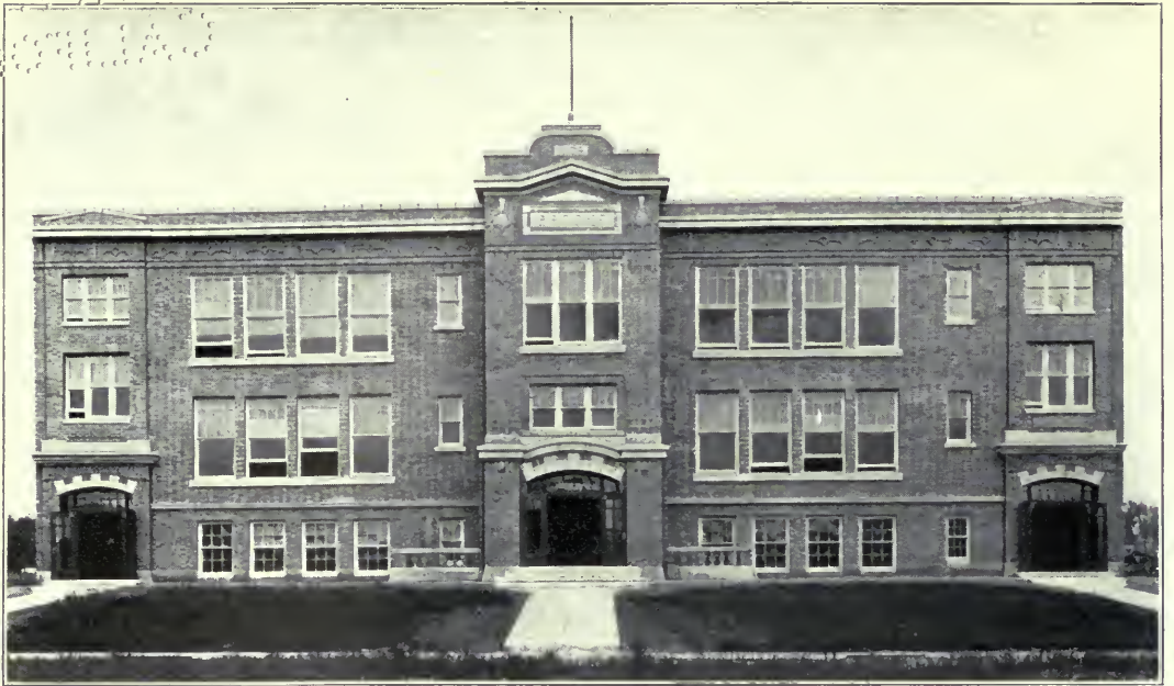
BROOKS SCHOOL, DES MOINES, IA. Wetherell & Gage, Architects
