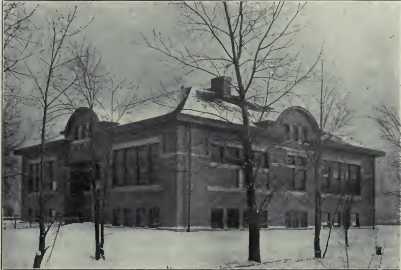
LINCOLN SCHOOL, OAK PARK, ILL. E. E. Roberts, Architect, Oak Park
