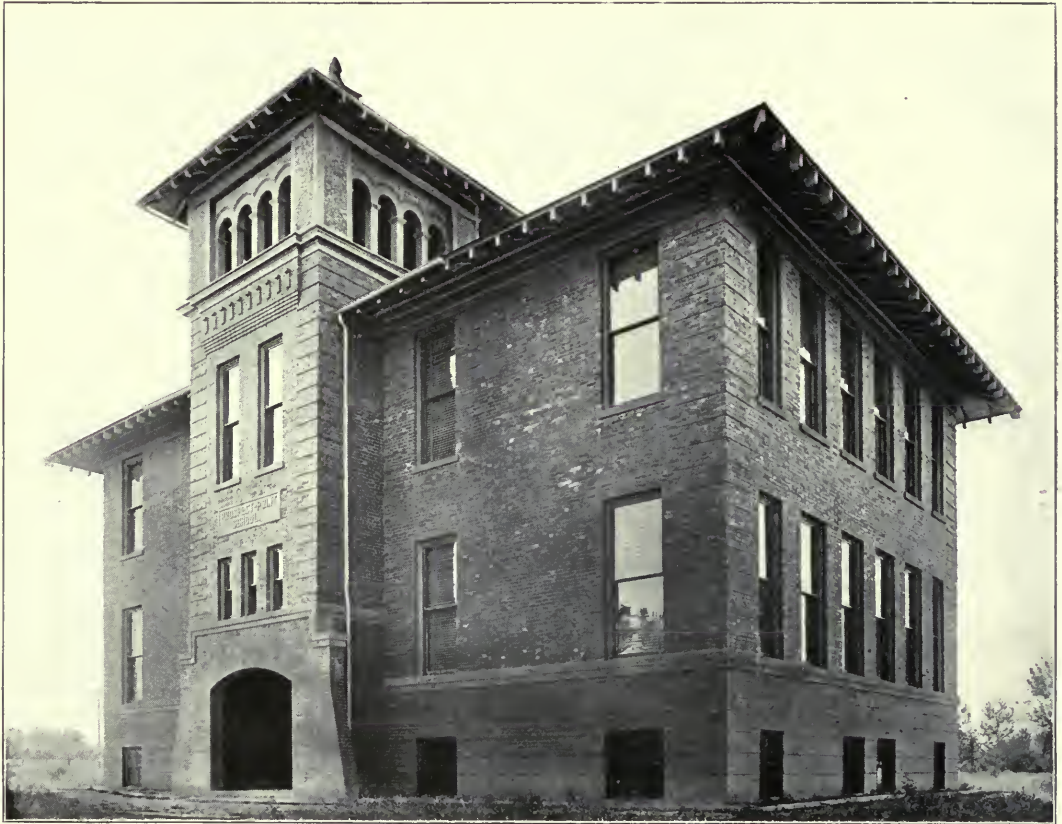
PROSPECT POINT CONSOLIDATED SCHOOL, NEAR WALLA WALLA, WASH.
