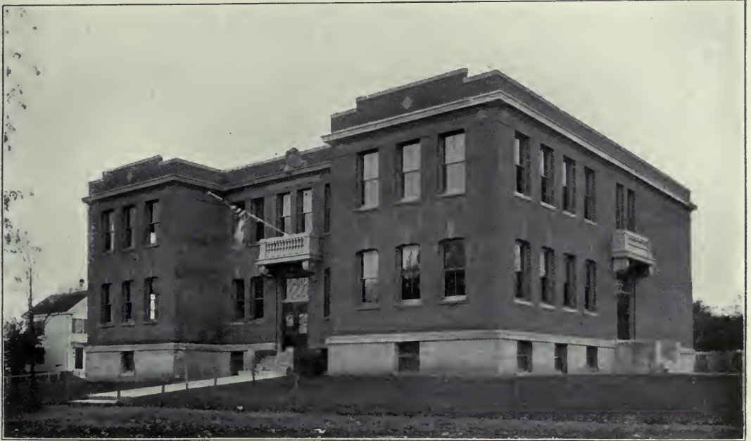
ALBERT CURRIER SCHOOL, NEWBURYPORT, MASS. Edward I. Wilson, Architect, Boston
