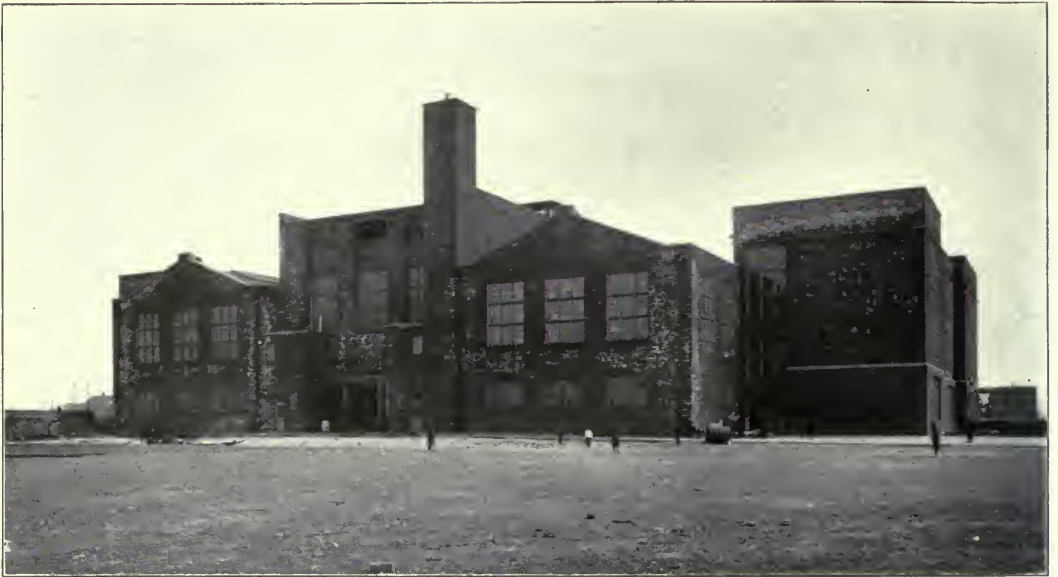
REAR VIEW, THE FROEBEL SCHOOL, GARY, IND. William B. Ittner, Architect. St. Louis, Mo.
