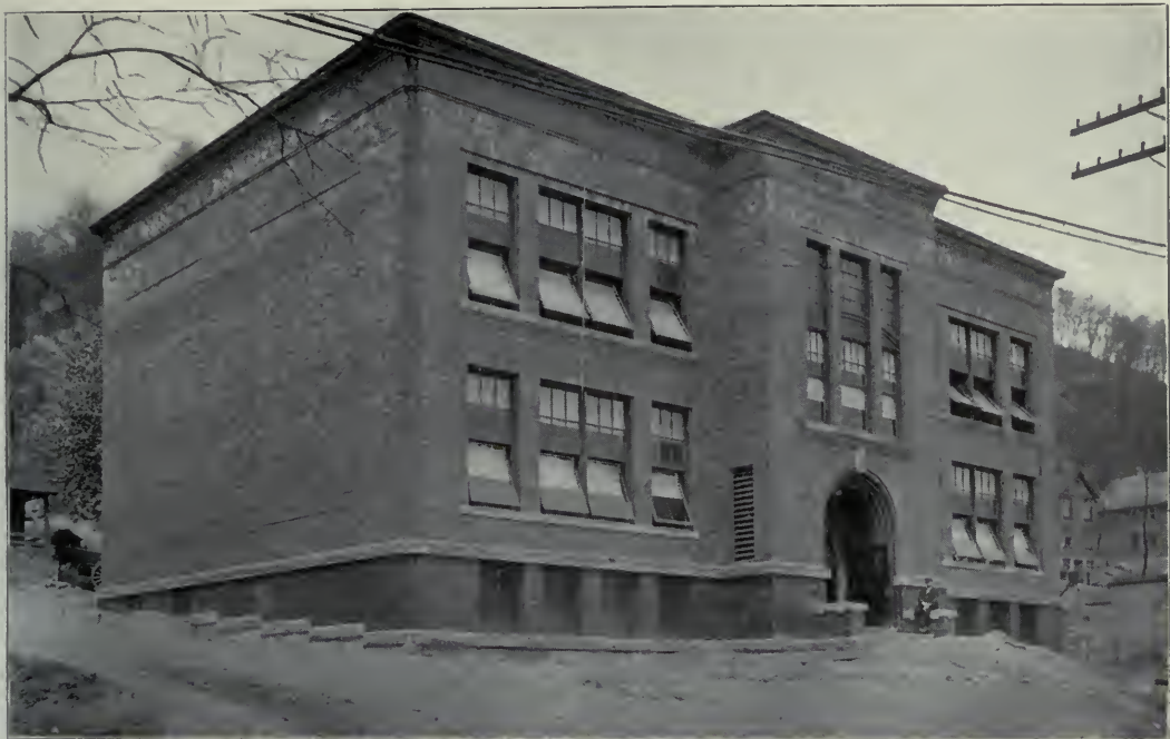
LOGSTOWN SCHOOL, WOODLAWN, PA. C. C. & A. L. Thayer, Architects, New Castle
