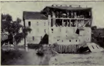
A flour-dust explosion wrecked this mill
