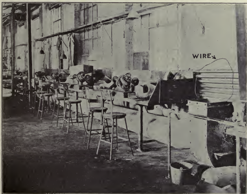
FIG. 15.—View of dust collecting system showing wire as found in fan following the explosion. Buffing brushes used can be seen on bench.
