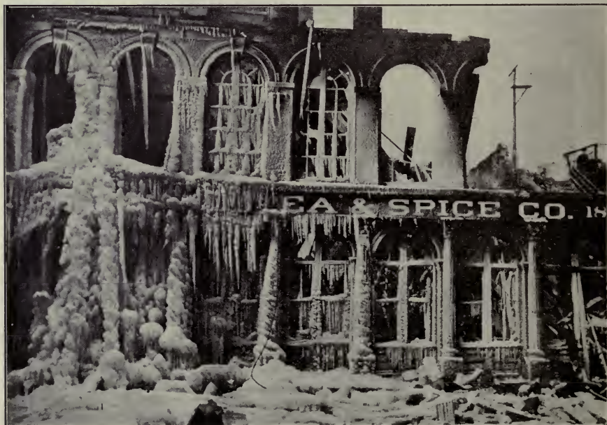
FIG. 14.—At extreme right can be seen bridge from which firemen were fighting the fire when the wall was blown out by explosion of spice dust.
