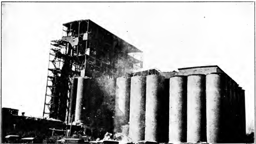
FIG. 13.—Explosion traveled from basement through man-lift tower to "texas" or top of elevator.
