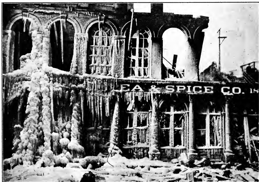
FIG. 14.—At extreme right can be seen bridge from which firemen were fighting the fire when the wall was blown out by explosion of spice dust.
