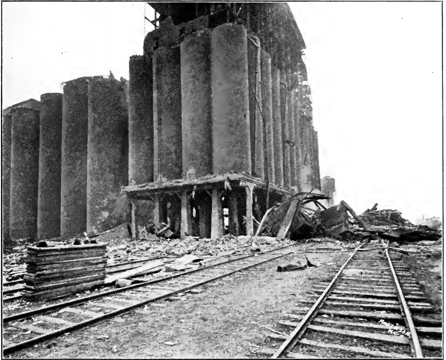
FIG. 12.—View showing violence of explosion and damage to working floor and shed. Explosion originated in basement.
