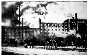
This large cereal plant was completely destroyed by fire following a dust explosion
