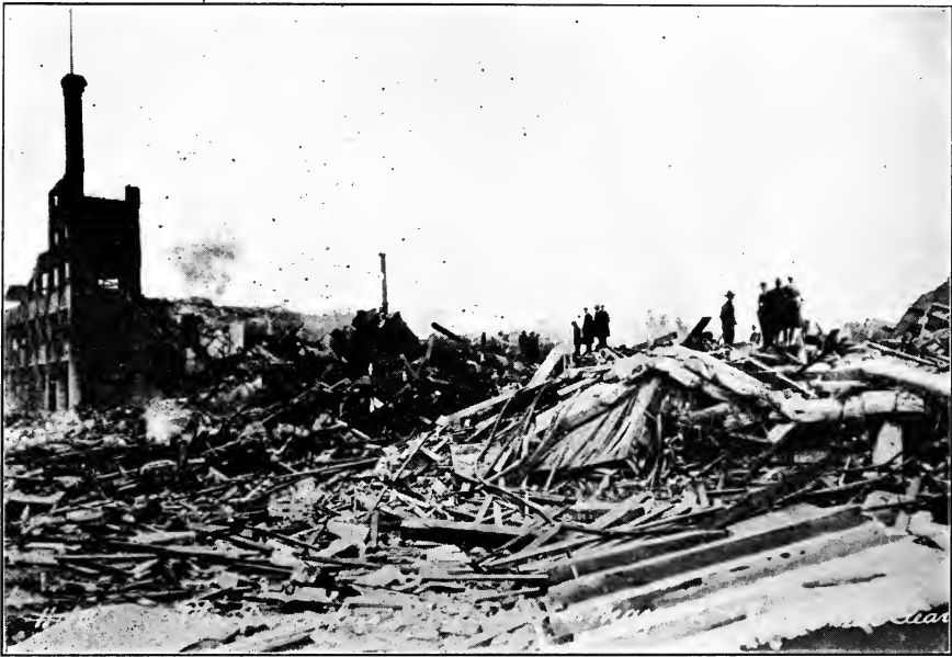
FIG. 9.—Extensive damage resulting from explosion of starch dust.
