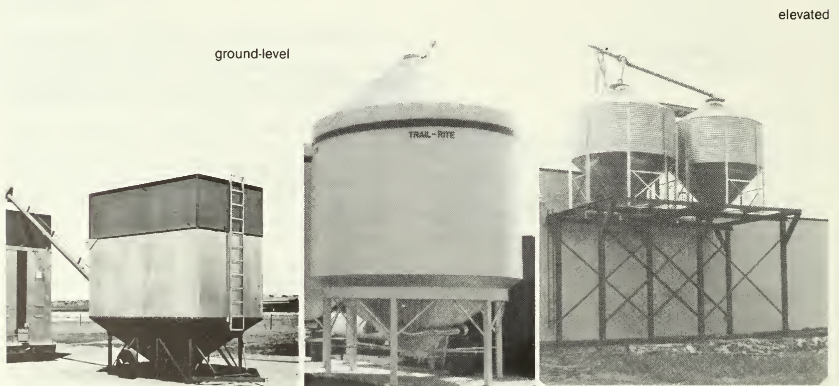
FIGURE 2 Structures to hold hopper-bottom bins
