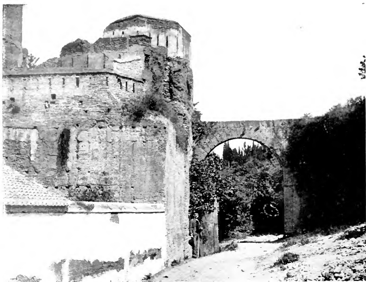
TOWER OF THE AQUEDUCT
