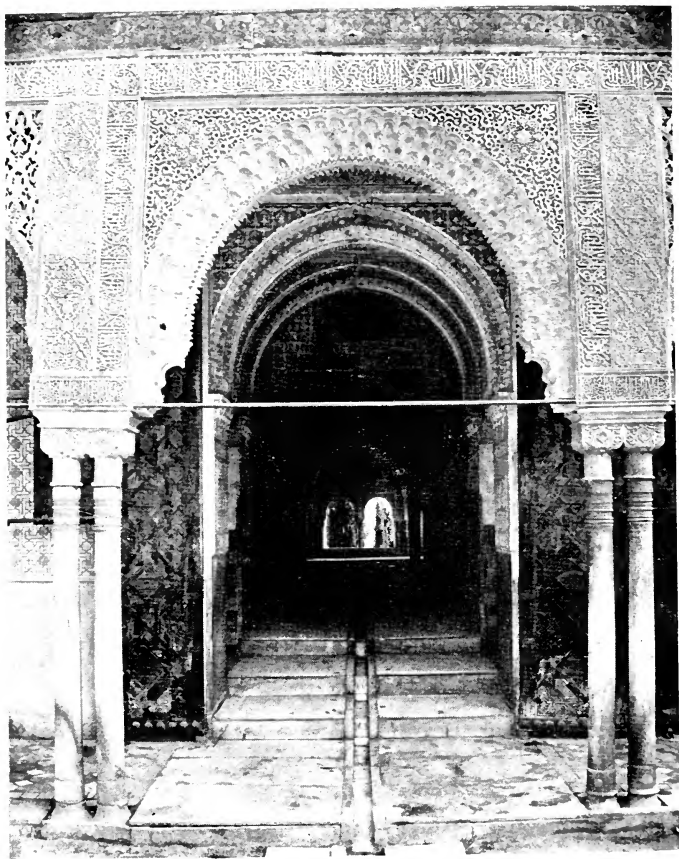
ENTRANCE TO THE HALL OF THE TWO SISTERS
