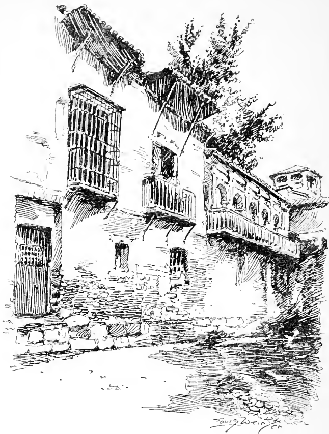
Exterior of an old House
