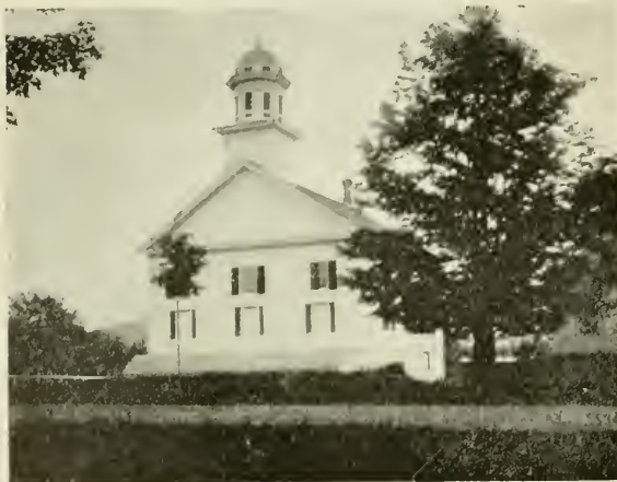
Methodist Church, at the Street.
