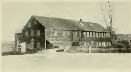
New Boston Electric Light Plant.
