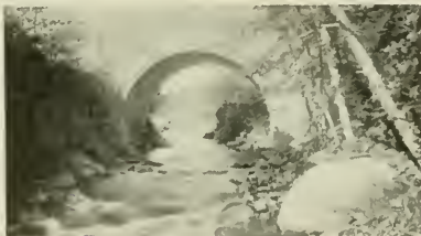
Stone Bridge from the South.
