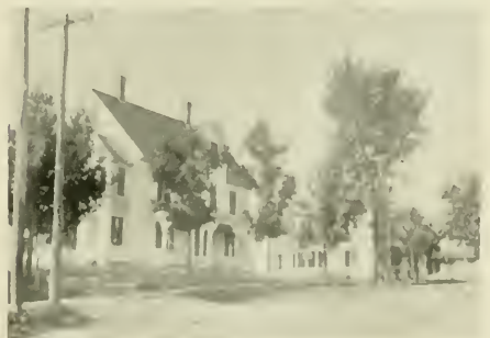
Part of Main Street, looking North.
