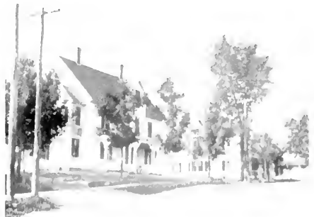
Part of Main Street looking North.
