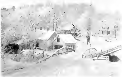
View Southwest from Valley Hall.
