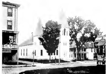
Methodist Church, Hillsborough Bridge.
