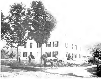
Residence of William Woodbury.
