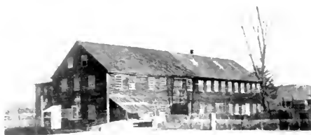
New Boston Electric Light Plant.
