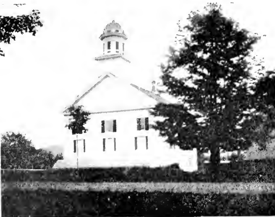
Methodist Church, at the Street.
