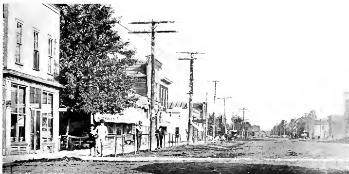
STERLING STREET, LOOKING NORTH.
