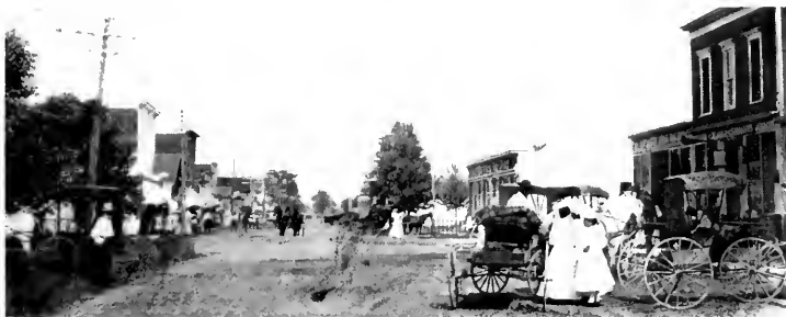
MAIN STREET, LOOKING EAST.
