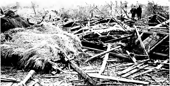
WRECKAGE OF BOWMAN BUILDING—MRS. BOWMAN WAS KILLED.
