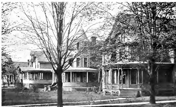
ON JEFFERSON STREET, SOUTH.
