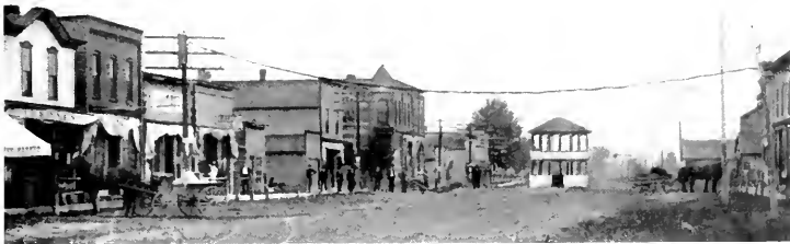
ROBISON STREET, LOOKING NORTH.
