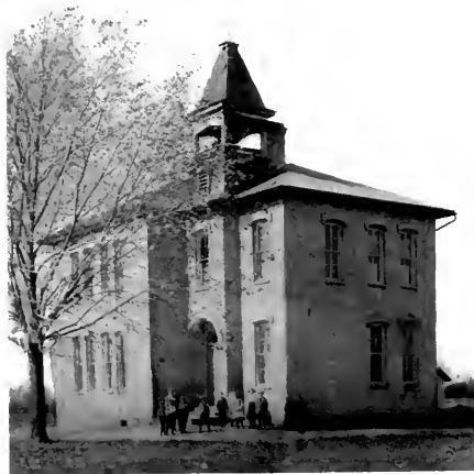
SUMNER'S SCHOOL BUILDING.
