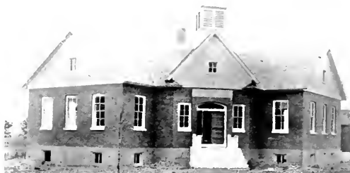
WHEELER'S SCHOOL BUILDING.
