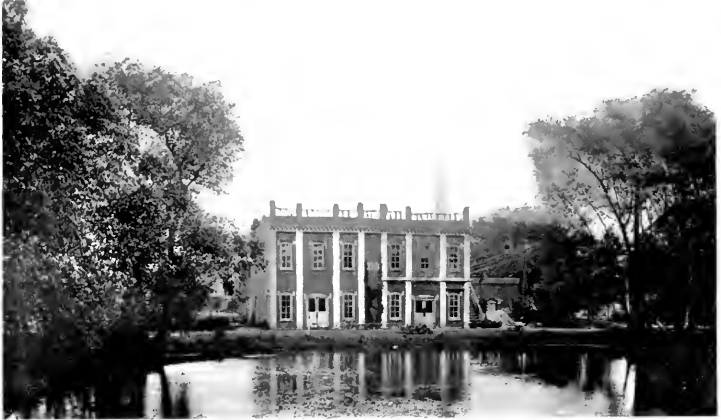
WATER AND LIGHTING PLANT.
