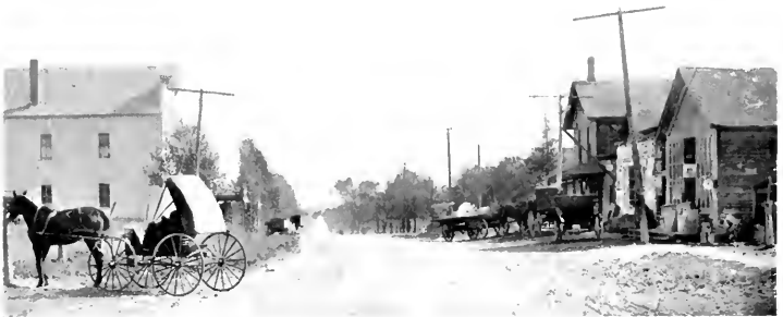
MAIN STREET, LOOKING EAST.
