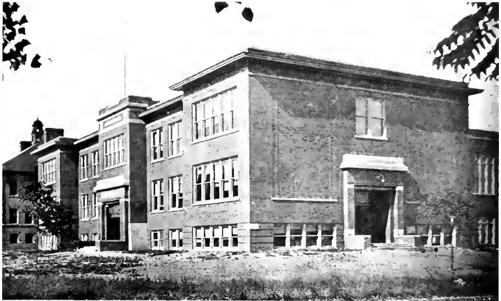
NEW $65,000 SCHOOL BUILDING—1912.
