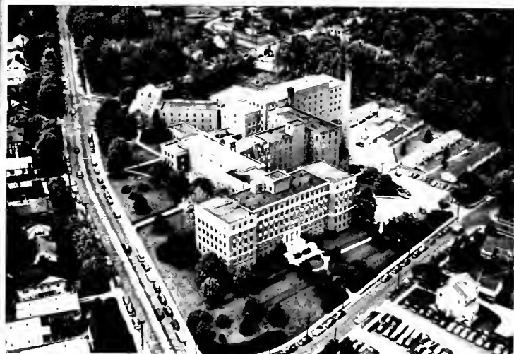
above: This photo, circa 1954, shows the 5th floor additions on both wings of the medical school (foreground), as well as the completed South Wing and smokestack (background).
