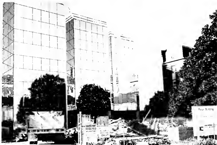
above: "Old Main", the original 1923 NCBH building, had to be torn down to make room for the Focus Building (now Watlington Hall). photo circa 1980.
