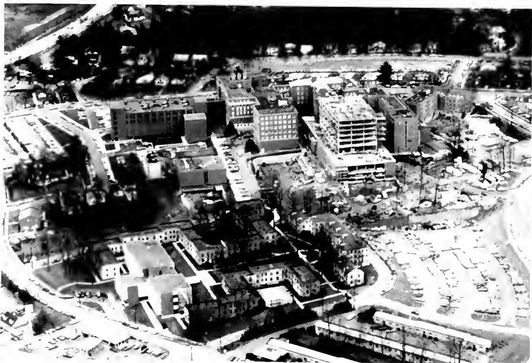
above: the Medical Center seen from the west in 1969 shows the Reynolds Patient Tower under construction while the Hanes Building has already been completed
