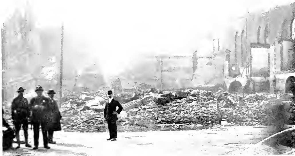
VIEW OF FIRE ZONE LOOKING WEST FROM ST CLAIR
