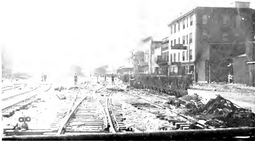
WASHOUT of TRACKS at UNION DEPOT
