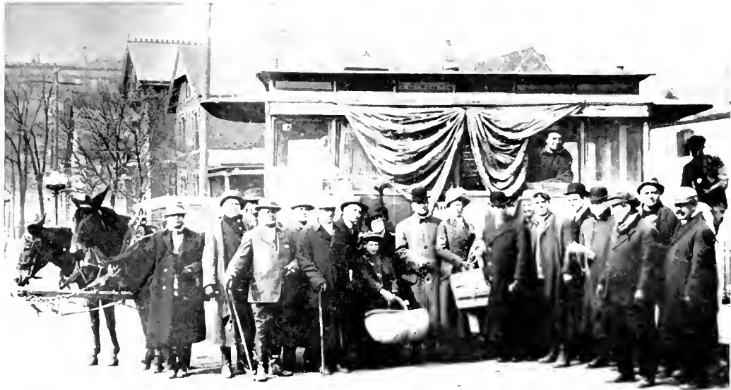
THE OLD MULE CAR IN SERVICE AFTER FLOOD
