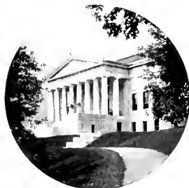
FRONT VIEW, HISTORICAL BUILDING
