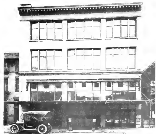
Pearl Street Entrance
