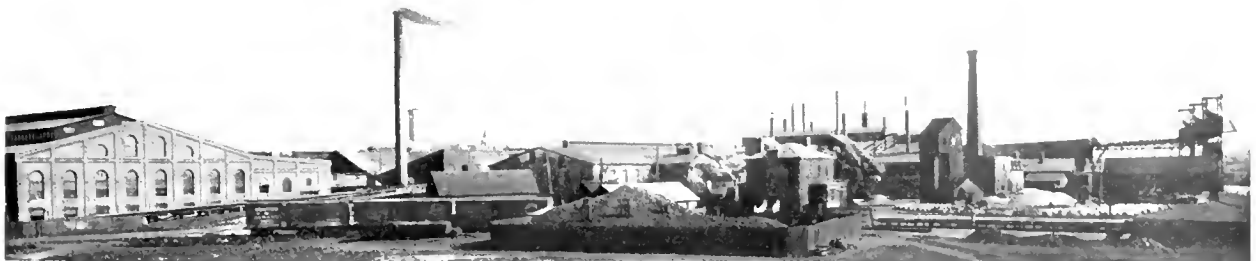
PLANT OF THE BUFFALO SMELTING COMPANY Manufacturers of Copper Ingots, Wire Bars, and Rolling Mill Cake
