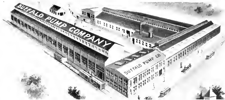
WORKS OF THE BUFFALO PUMP COMPANY, NORTH TONAWANDA
