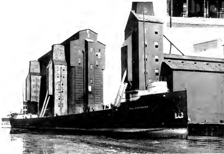
BUFFALO HARBOR One of Buffalo's twenty-three elevators. Lake steamer unloading
