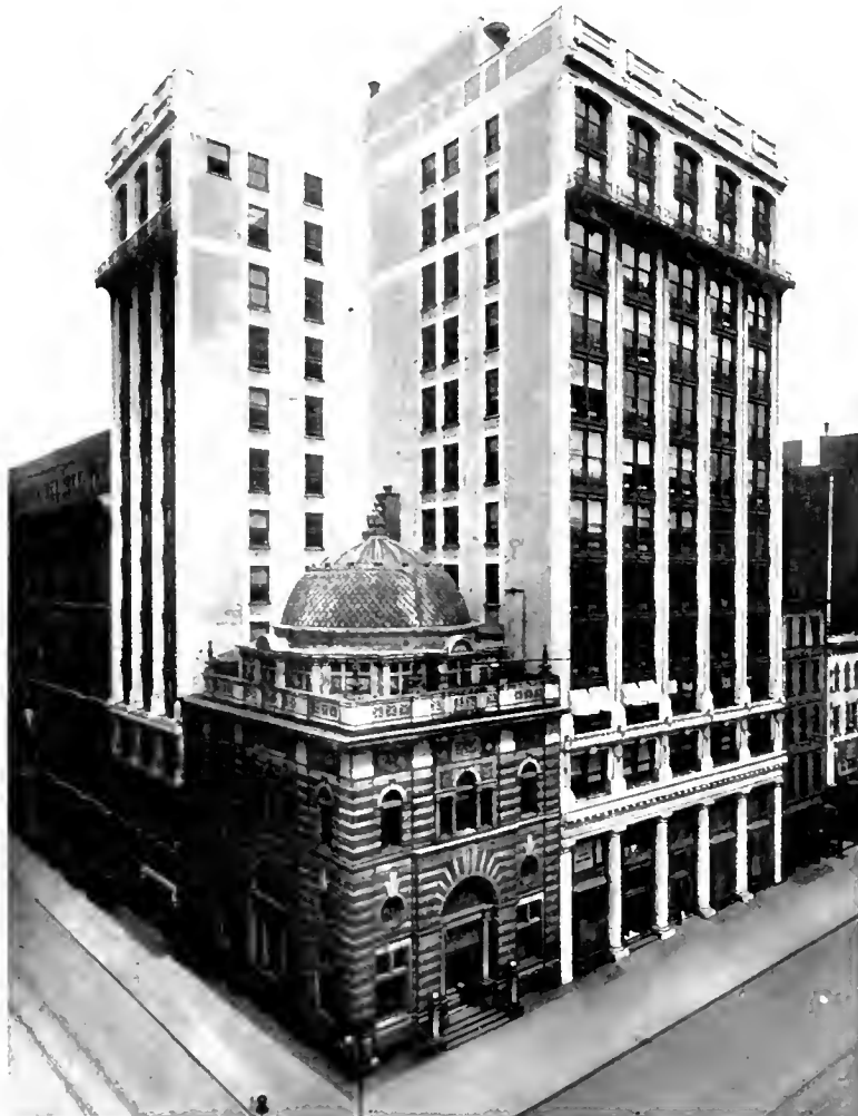
BUFFALO CHAMBER OF COMMERCE BUILDING
