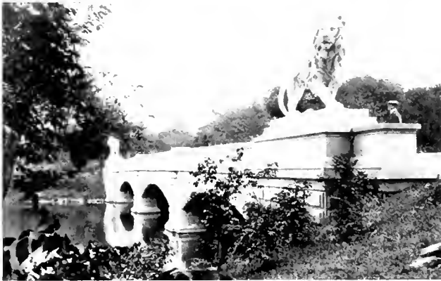
DELAWARE PARK BRIDGE
