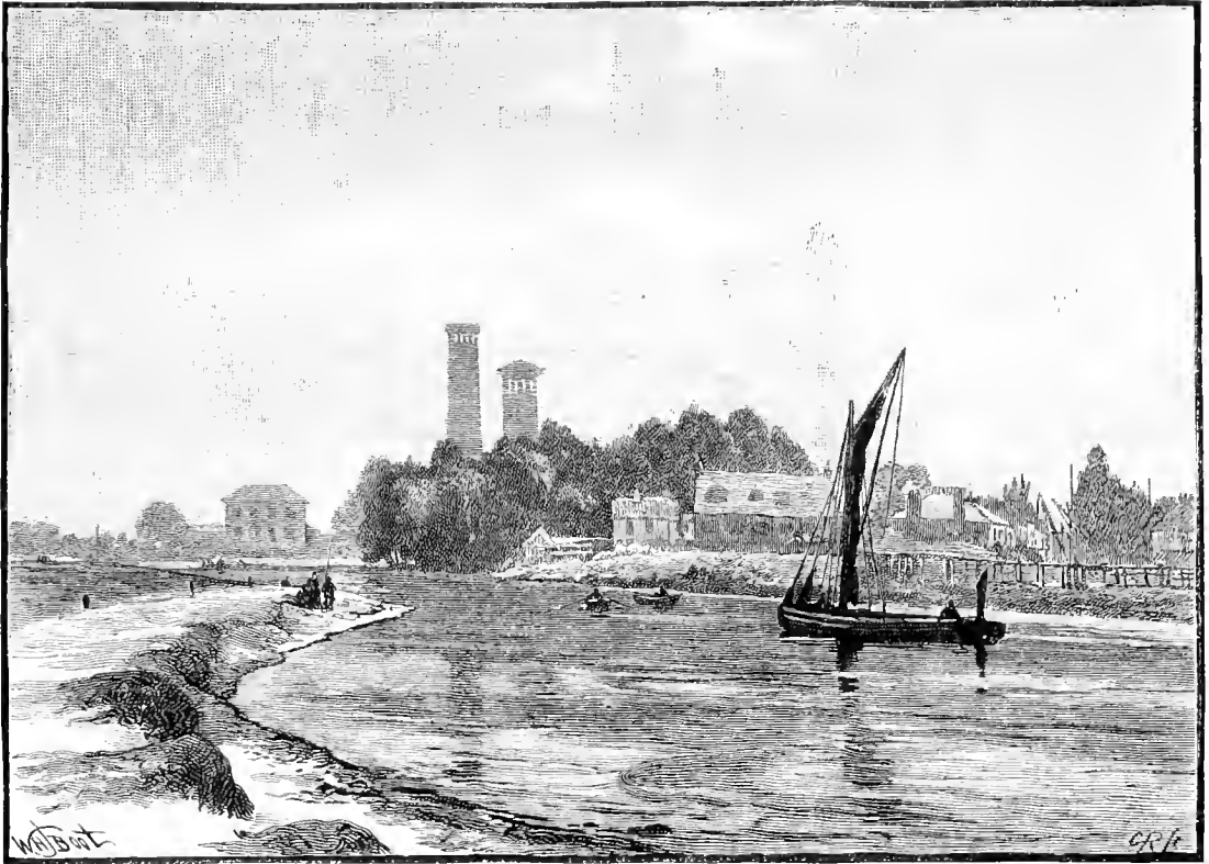
AT LEA BRIDGE.
