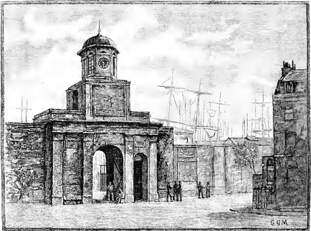
ENTRANCE TO THE EAST INDIA DOCKS.
