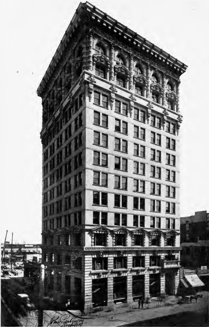
UNION TRUST BUILDING. JOHN PARKINSON, ARCHITECT.
