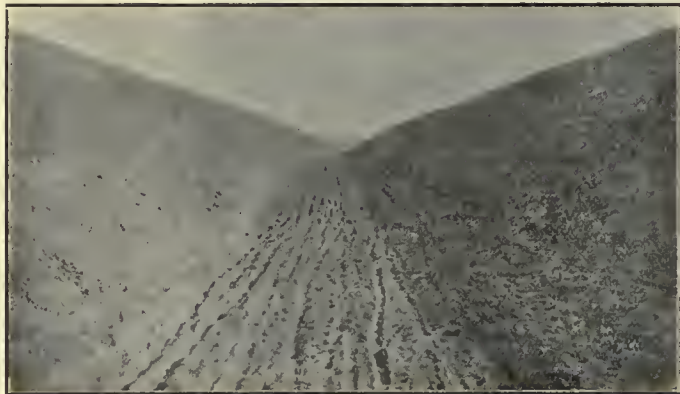
A PORTION OF THE COMPLETED DITCH
