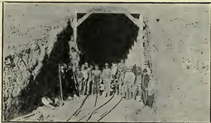
ONE OF THE TUNNELS WHICH WILL BE LINED WITH CONCRETE, THROUGH WHICH THE WATER PASSES
