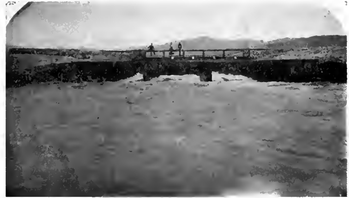
WASTE-GATE OF THE RESERVOIR OF THE LOVELOCK LAND & DEVELOPMENT CO. Through this passes all waste or water not needed by the Company for their purposes.
