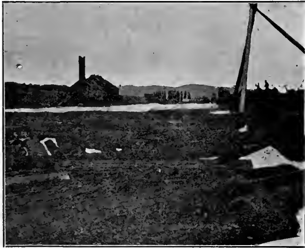
RENO MILL AND LUMBER CO. MILL AT LOYALTON
