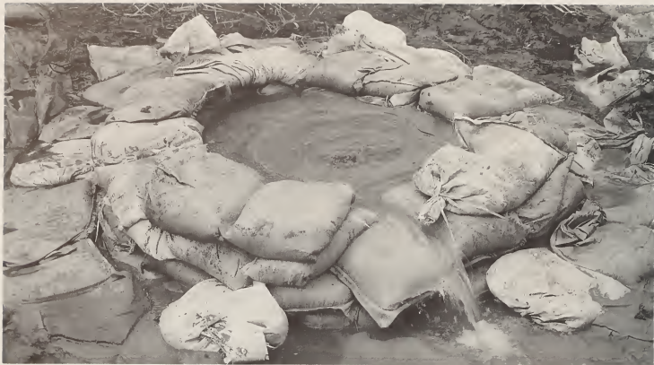
25 Pike County: Sand boil at the foot of the Sny Island levee. Sandbag ring dike prevents loss of piped sand but lets water flow away, reducing water pressure under the levee (July 21, 1993).
