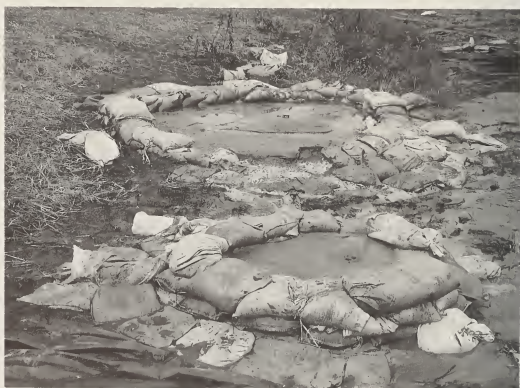
25 Pike County: Sand boil at the foot of the Sny Island levee. Sandbag ring dike prevents loss of piped sand but lets water flow away, reducing water pressure under the levee (July 21, 1993).
