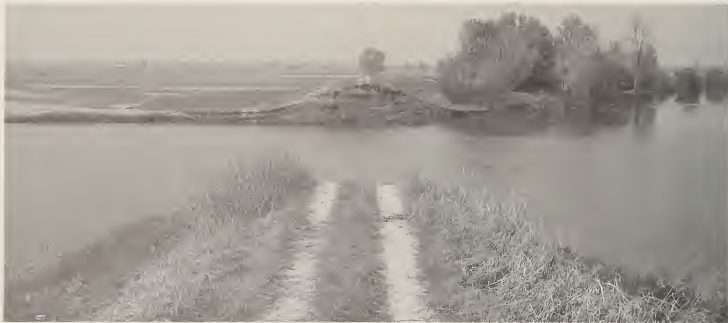
30 Randolph County: Looking northward across the levee breach in the Kaskaskia Island levee. (Figure 31 shows the depth of scour through this breach.) The Mississippi River channel is to the right beyond the range of the photo. (October 13, 1993).
