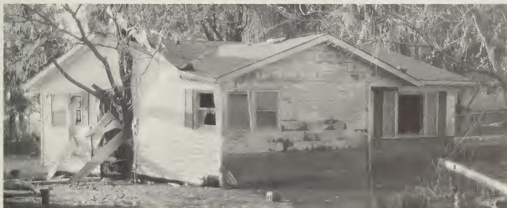
2 Monroe County: Flood water rushing through the town of Valmeyer lifted this house off its foundation and carried it until it collided with a tree (October 12, 1993).
