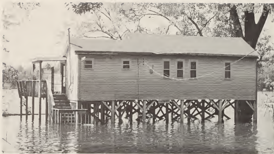
3 Adams County: High water came up to the windows of this house on stilts along the Mississippi River near Quincy. Oily film of silt and clay covers the lower half. Although the house stayed high and dry during other floods, it was not safe from the flooding in 1993, which exceeded the design height for flood protection (August 25, 1993).
