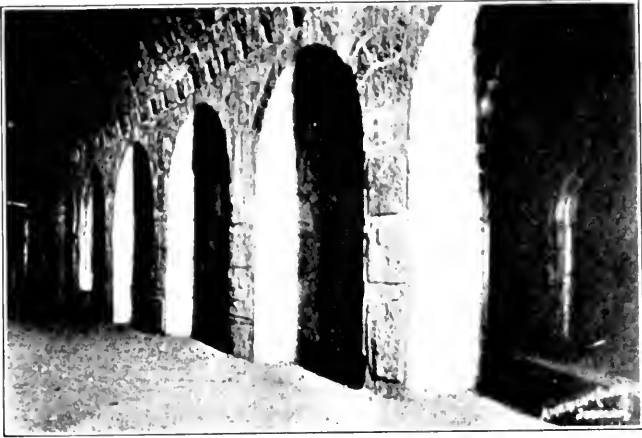
Substructures of Temple Area
