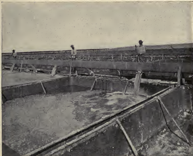
FIG. 13.—Dissolving nitrate from crushed caliche.
