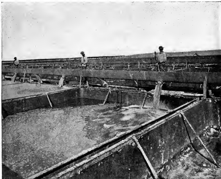
FIG. 13.—Dissolving nitrate from crushed caliche.
