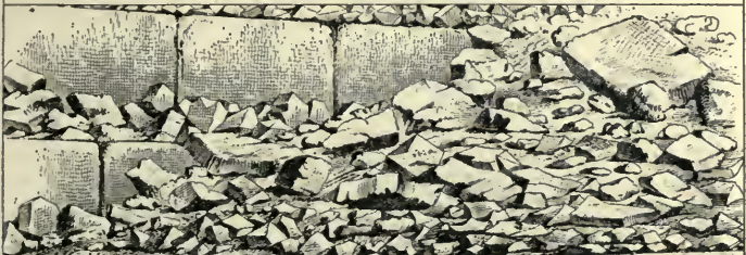
EXAMPLE OF THE CASING-STONES OF A PYRAMID, SUPER-POSED. ON THE RECT-ANGULAR MASONRY COURSES: FROM A PHOTOGRAPH BY P.S. OF THE SUMMIT OF THE 2 d PYR.
