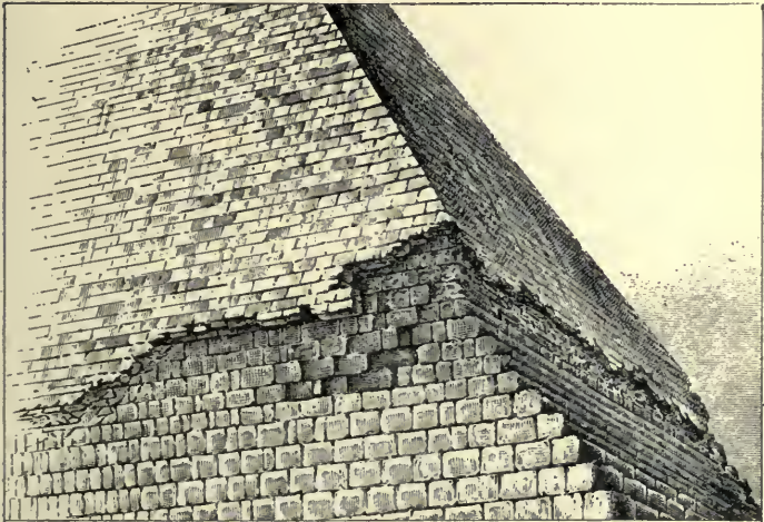
EXAMPLE OF THE CASING-STONES OF A PYRAMID, SUPER-POSED. ON THE RECT-ANGULAR MASONRY COURSES: FROM A PHOTOGRAPH BY P.S. OF THE SUMMIT OF THE 2 d PYR.
