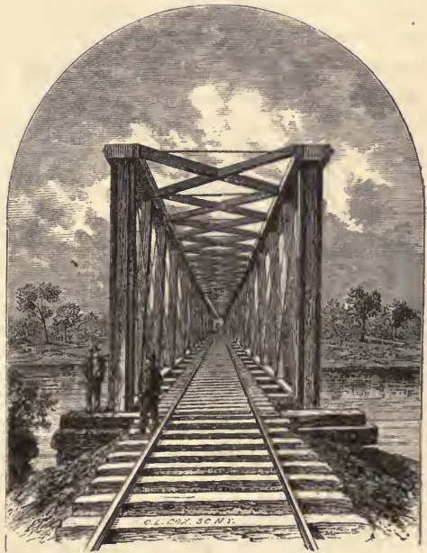
Bridge across the North Fork of the Canadian River, Indian Territory (M., K. & T. Railway).
