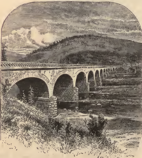
Cumberland Viaduct, Maryland.
