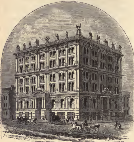
The St. Louis Life Insurance Company's Building.
