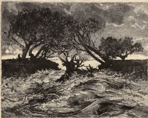
A Crevasse in the Mississippi River's Banks.
