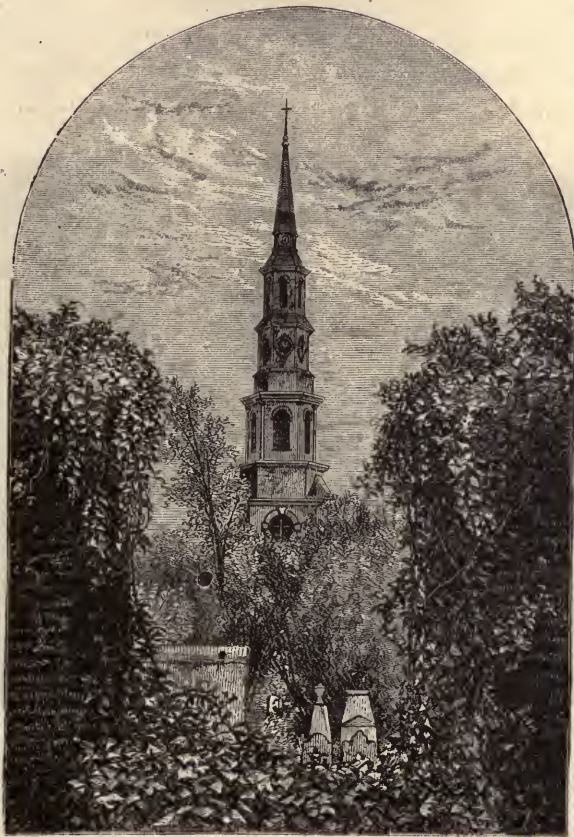
The Spire of St. Philip's Church—Charleston.
