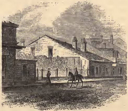
"Some aged private dwellings, rapidly decaying."
