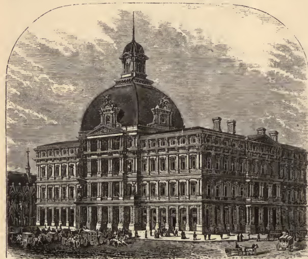
The new Post-Office and Custom-House in construction at St. Louis.
