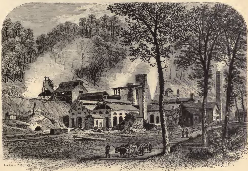
The Rockwood Iron-Furnaces—Eastern Tennessee.
