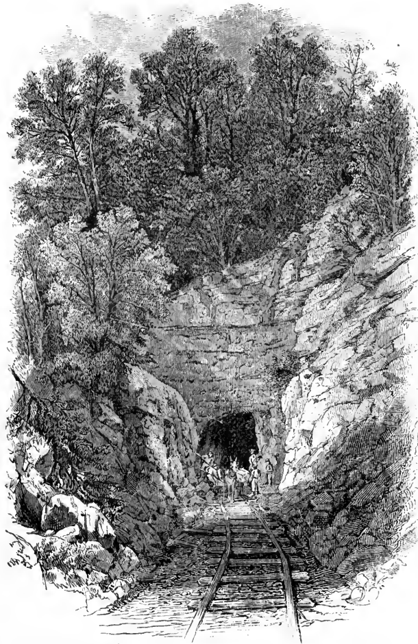
The Eastern Portal of Second Creek Tunnel, Chesapeake and Ohio Railroad.
