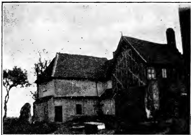
No. 1. North Side.
