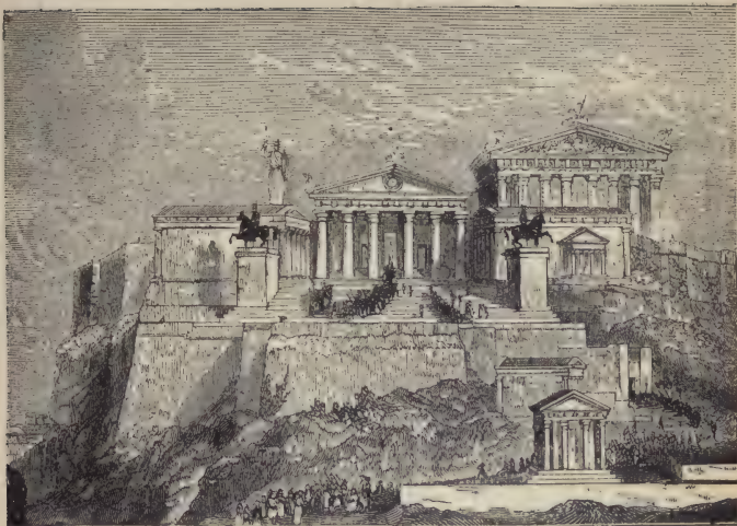
RESTORATION OF THE WEST END OF THE ACROPOLIS.*
