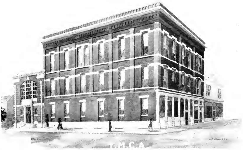
Y. M. C. A. BUILDING, XENIA. Showing proposed new Gymnasium in rear.
