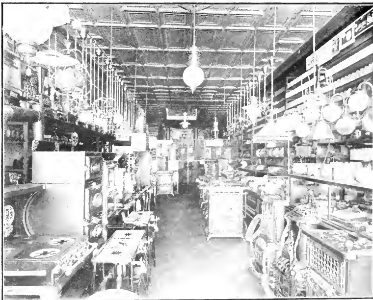
ROBERT H. SNEAD, 21 GREEN ST. PHOTO BY THE AUTHOR Natural Gas Fitting and Plumbing. Gas and Electric Supplies.
